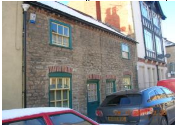
Figure 3.140: Frontage of 31 & 33 Norfolk Street.
