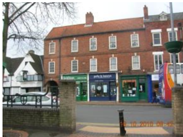
Figure 3.16: 130-132a Bridge Street, as viewed from Market Place.
