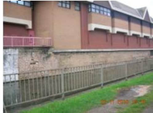
Figure 3.106: View of part of earlier building on north side of canal.
