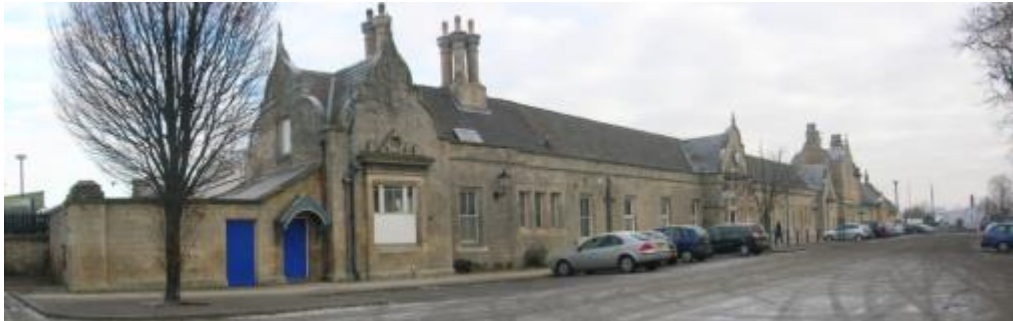
Figure 3.160: View of original station building from south west.
