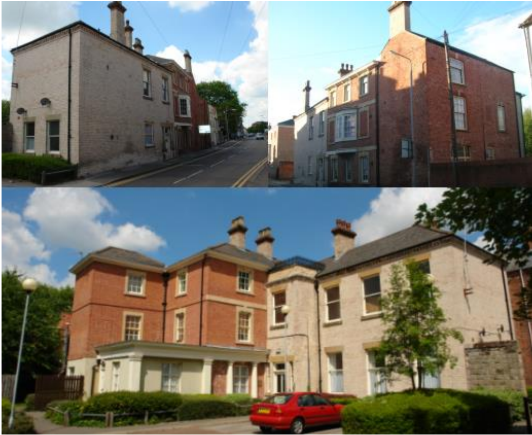
Figure 3.23: Park House, Park Street, from south east (top left), from north east (top right) and from south west (bottom). The three distinct phases of construction can be seen together along the frontage.
