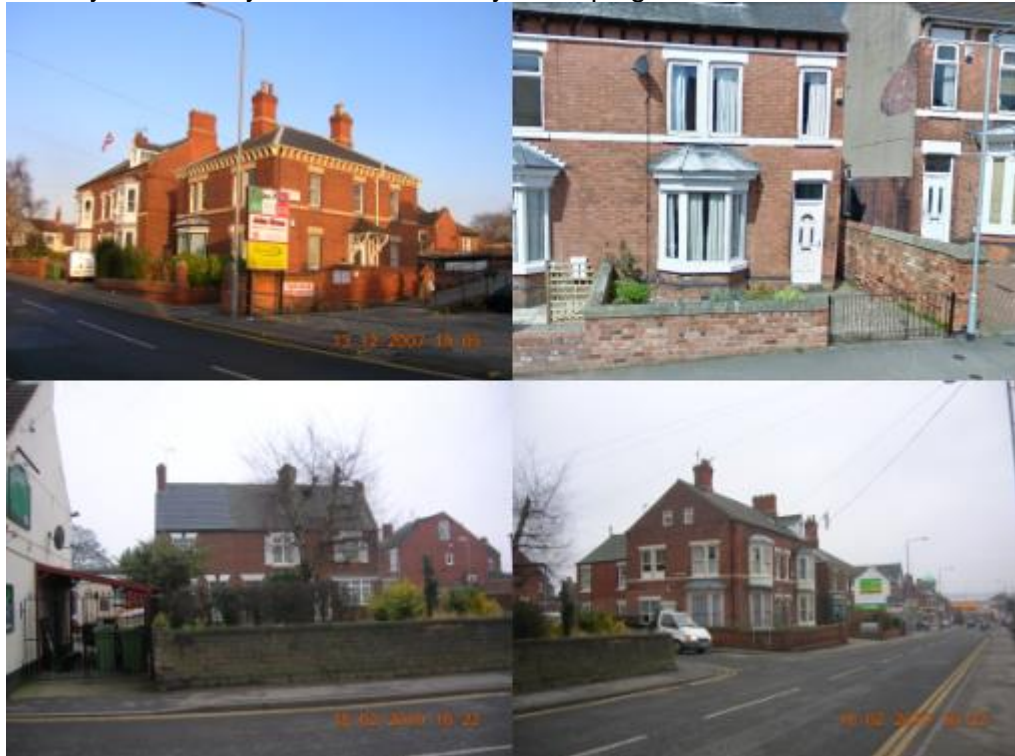
Figure 3.177: Top left: Brick boundary walls with stone and clay coping at 76 Carlton Road and 15 Sherwood Road (top right, source: Google Maps, 2010); Bottom left: Late 18 th /early 19 th century stone boundary wall at junction of Carlton Road with Sherwood Road; Bottom right: The same stone wall (left) with brick wall and stone coping around 80 Carlton Road (right).
