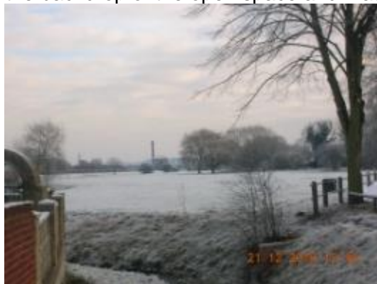
Figure 3.97: View of Bracebridge Pumping Station from Priorswell Road, looking eastwards.
