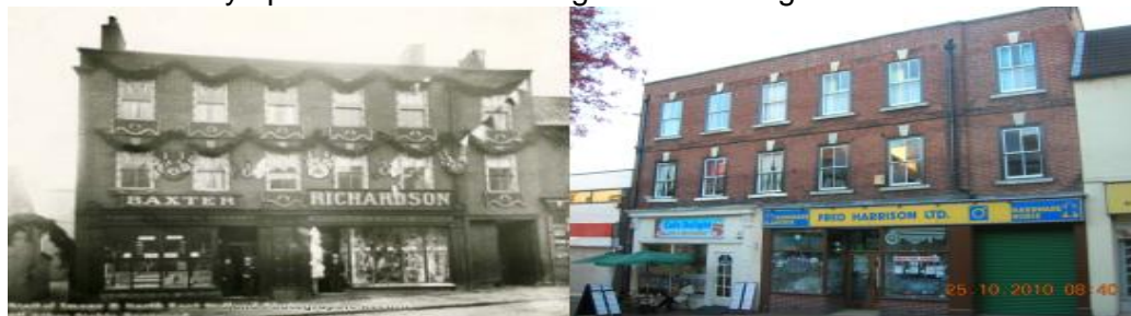
Figure 4.1: 79 & 81 Bridge Street, in 1891 (left) and present day (right). Originally a house built in the late-18 th century, with the shop fronts added in the late-19 th century. Whilst elements of the 19 th century shop fronts still survive on No.79, the frontage on No.81 is of a traditional shape although is of modern materials. The signage on both frontages is excessively large and appears unsympathetic with the building. The roller shutter (bottom right) also appears intrusive on the building – timber shutters/gates would be preferable. Source: www.picturethepast.org.uk , 2010.
