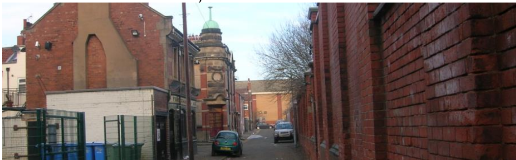
Figure 3.135: View northwards along Beaver Place, towards former Gas Offices (centre).
