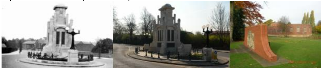
Figure 3.79: Listed War Memorial from 1950 (left) and present day (centre). Former Victoria Hospital War Memorial in grounds of library (right). Source: www.picturethepast.org.uk , 2010.
