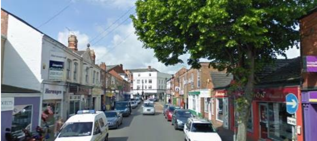
Figure 3.59: View westwards along Ryton Street, towards Burton building (distant centre). Source: Google Maps, 2010.
