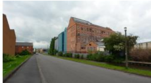
Figure 3.102: View along Canal Road from east, looking west towards Smith's Flour Mill (right).
