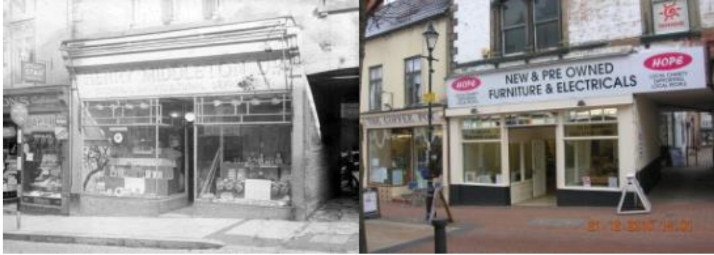
Figure 4.2: 87 Bridge Street, in 1939 (left) and present day (right). The majority of this late 18 th /early 19 th century building's shop front has been replaced, although traditional materials are used, albeit with a wider doorway. However, the signage panel is overly large and also covers the archway adjacent. Potential improvements could include the re-installation of the cornice and pilasters and the re-sizing of the signage, to more closely resemble that which existed in the 1930s. Source: Bassetlaw Museum, 2010.
