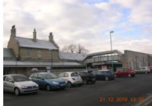
Figure 3.166: View of both platforms and connecting iron footbridge, from north east.
