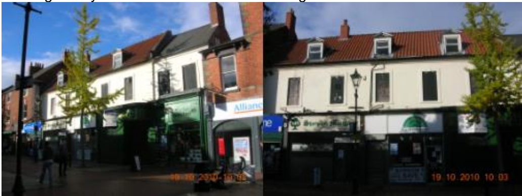
Figure 3.22: Views of frontage to 60-66 Bridge Street
