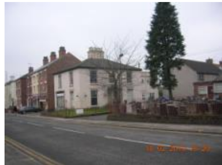
Figure 3.173: View of 45 Carlton Road, from north east.
