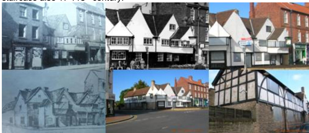
Figure 3.11: Top row: East elevation of Ship Inn from c.1930, 1970 and 2010; Bottom row: Ship Inn from south east in 1848 (left) and present day (centre); Bottom Right: Ship Inn from south west. Image sources: www.picturethepast.org.uk , (2010) and Victorian Worksop, (Jackson, M. 1992).
