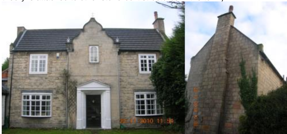
Figure 3.111: Left: Frontage of 38 Church Walk; Right: West elevation, facing rear garden of No. 36.
