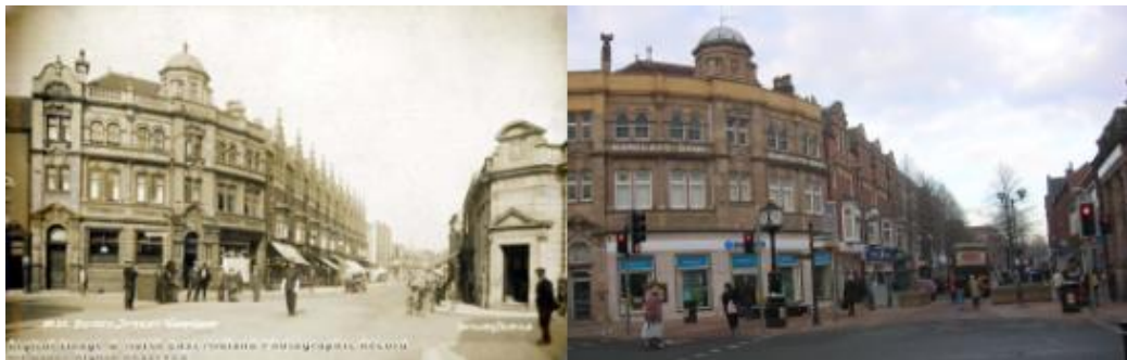
Figure 4.6: Barclays Bank, 2 Newcastle Avenue in 1920 (left) and present day (right). Several elements of the Barclays Bank building have been lost over time, including the decorative parapet above the second floor and most of the ground floor frontage. This appears to have been completely replaced in the 1950s/60s. Modern fascia signage with internal illumination appears as an intrusive feature on an otherwise historic building. Source: www.picturethepast.org.uk , 2010.
