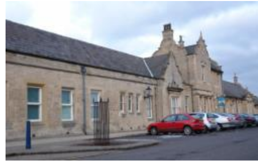
Figure 3.159: View of frontage of Worksop Railway Station from south west.
