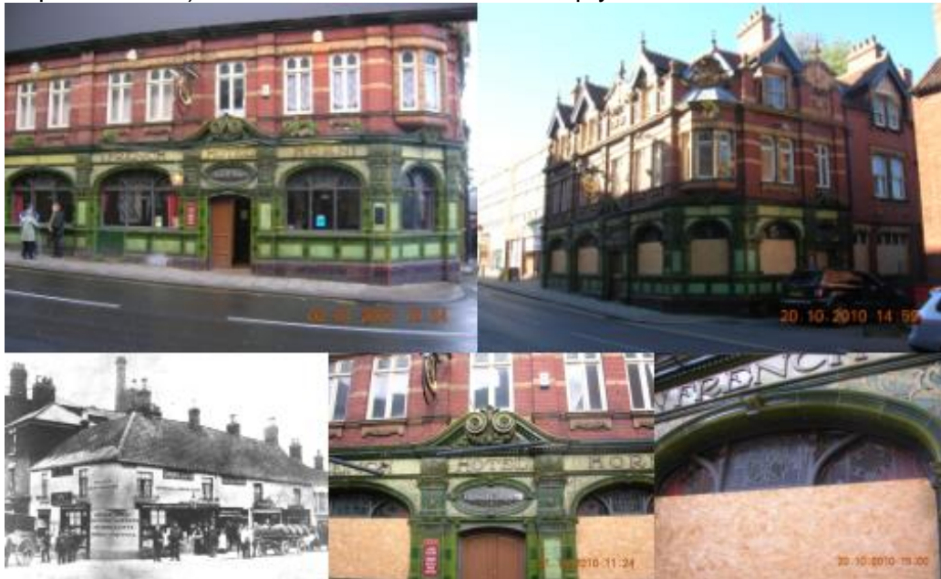
Figure 3.33: Top left: French Horn in 2007 prior to closure. Top right: Present day. Bottom left: Former Hooson Bros. store to west, 1910 (source: www.picturethepast.org.uk , 2010). Bottom centre: Oval overhead above front entrance. Bottom right: Arched window openings with tracery and stained glass designs.
