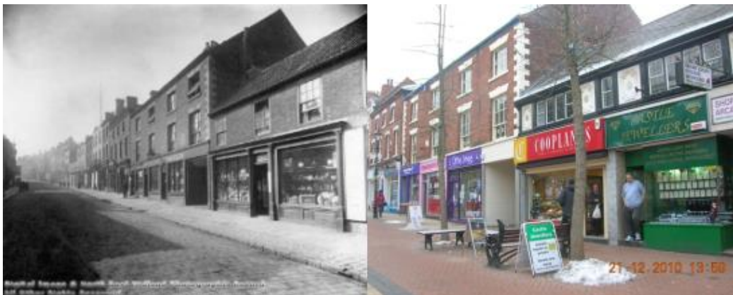
Figure 4.4: 70 & 70A Bridge Street in c1890 (left) and present day (right). Although the first floor was re-clad in the mid-20 th century, the division of the ground floor into two units has resulted in the loss of the historic 19 th century shop front with stallrisers, pilasters and a cornice. Both current frontages also contain large fascia signs that dominate the main aspect of the building. Source: www.picturethepast.org.uk , 2010.
