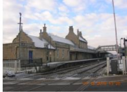
Figure 3.164: View of Railway Station from north east.
