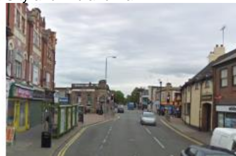
Figure 3.154: View eastwards along Newcastle Avenue, towards the bank (centre left). Source: Google Maps, 2010.
