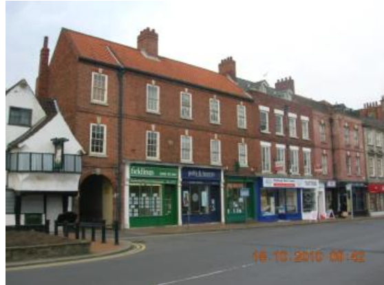
Figure 3.17: Georgian buildings on Bridge Street, opposite Market Place.
