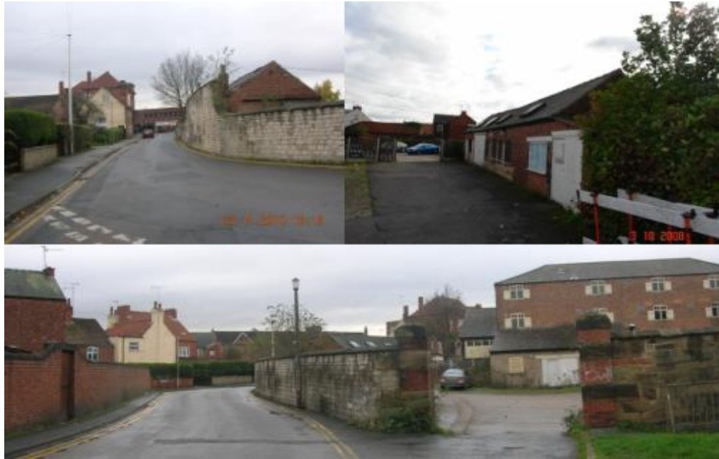
Figure 3.110: Top left: Stone boundary wall to south of former depository and canal cottage; Top right: Former blacksmiths' forges attached to boundary wall; Bottom: View of boundary wall and entrance to east of former depository, off Canal Road.
