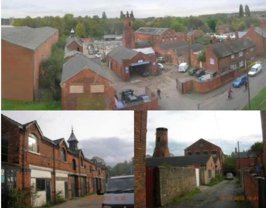
Figure 3.120: Top: View of Corporation Yard from upper floor of Smith's Flour Mill to north; bottom left: View of workshops with cupola-style ventilator on roof in eastern part of site, from north west; Bottom right: View of water tower/hose tower from north, looking south.
