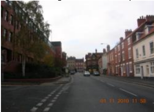
Figure 3.52: View westwards along Potter Street towards Bridge Street, with the French Horn (centre right) particularly prominent).
