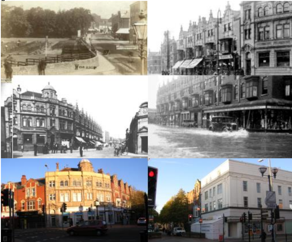
Figure 3.35: The Arcade site in 1900 (top left); 1903, south elevation (top right); 1930, south east corner (centre left), 1932 during a flood, north east corner (centre right); modern day, south east corner (bottom left) and north east corner (bottom right). Sources: www.picturethepast.org.uk and Bassetlaw Museum, 2010.
