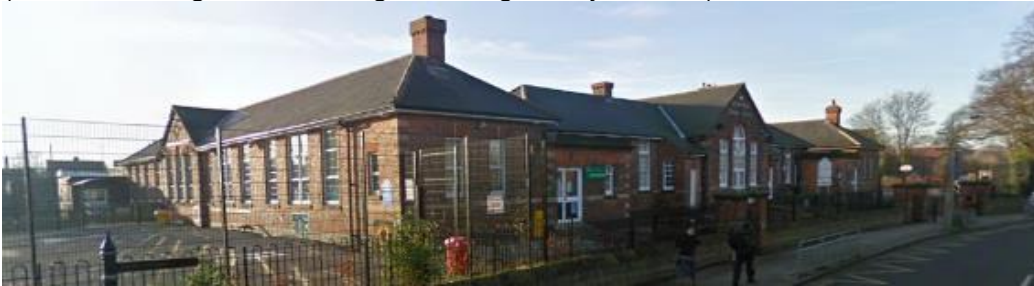
Figure 3.75: View of former Worksop Central School from north east (source: Google Maps, 2010).
