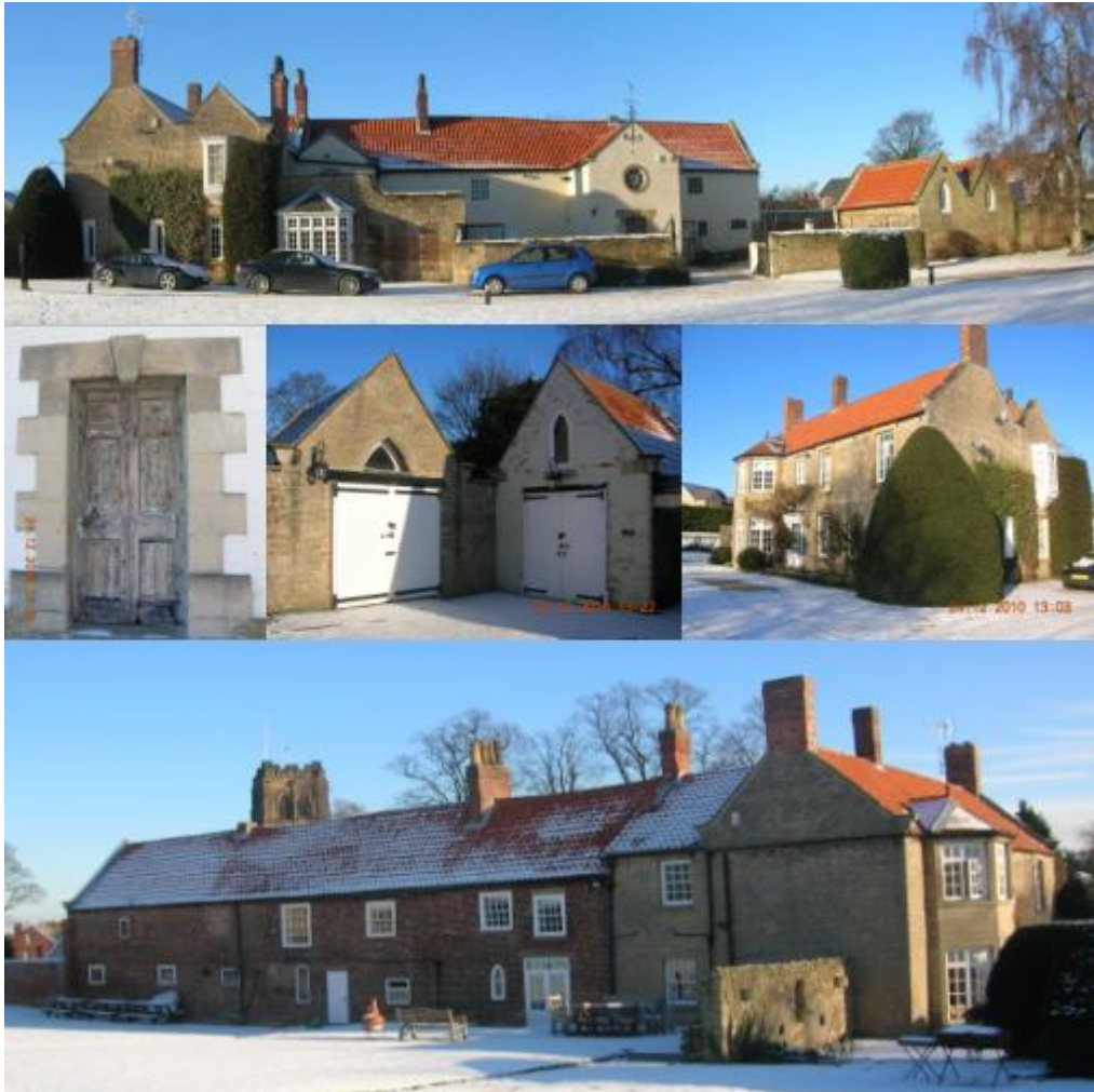
Figure 3.137: Views of Park Cottage from east (top) and south west (bottom); Doorway believed to be associated with James Gibbs (centre left); South elevation of building (centre right); gothic design of outbuildings (centre).
