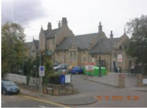
Figure 3.163: View of Railway Station from south east.
