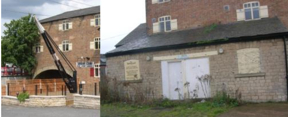
Figure 3.108: Left: Lifting winch/crane to west of former depository. Right: Magnesian Limestone lean-to extension to east of former depository.
