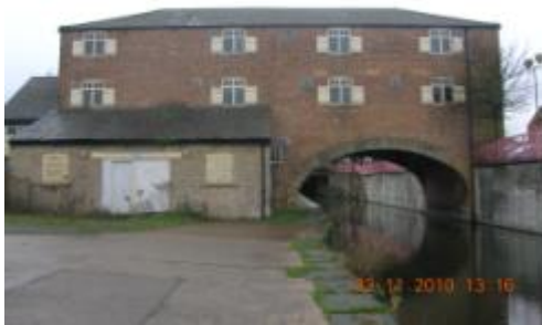
Figure 3.105: Rear of former canal depository, viewed from east.
