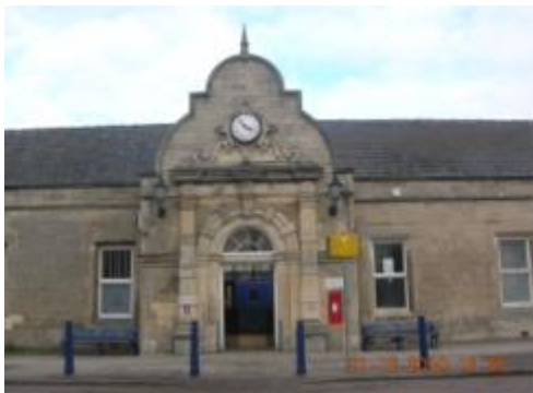
Figure 3.161: View of main entrance, from south.
