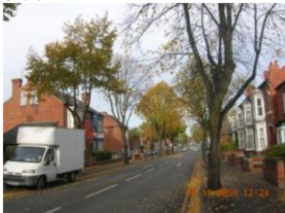
Figure 3.63: View along late 19 th Watson Road from south, looking north towards junction with Newcastle Street/Memorial Avenue
