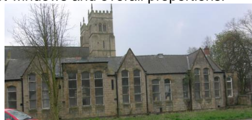
Figure 3.72: Church Hall, north elevation.
