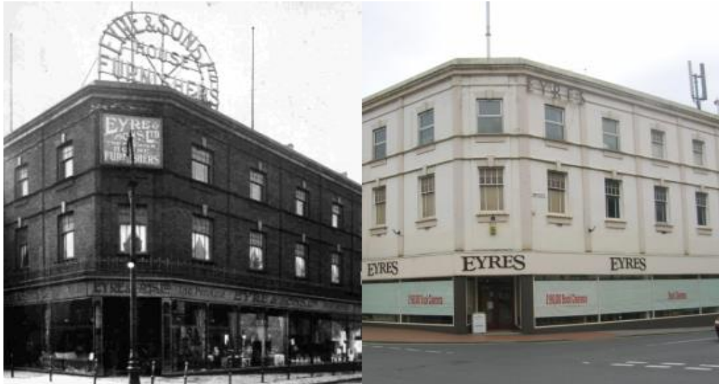
Figure 4.5: Eyres, Park Street, in 1910 (left) and present day (right). Other than the painting of the exterior in the mid-20 th century, this building has changed very little since first constructed. However, the loss of first floor transom windows and replacement with UPVC harms the significance of the building. In addition, the replacement of the angled signage (and associated decorative ironwork) with flat signage is also detrimental to the character of the building and its setting. Source: www.picturethepast.org.uk , 2010.
