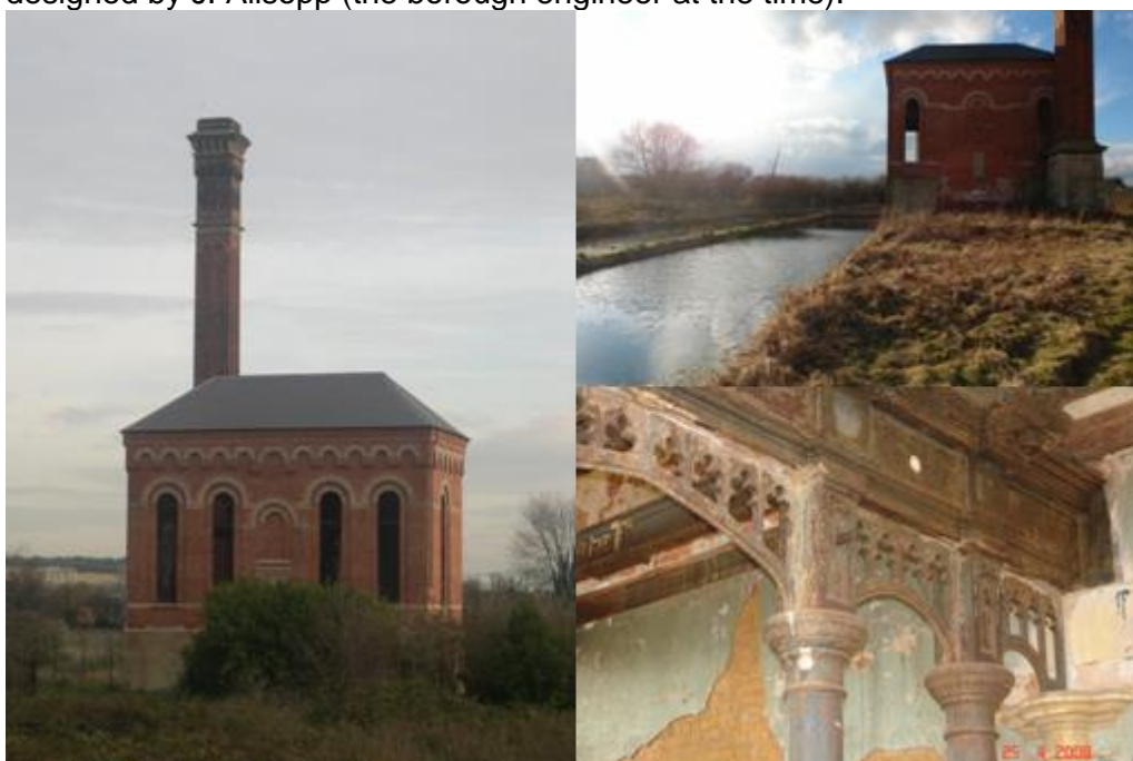
Figure 3.84: Views of Bracebridge pumping station from west (left) and east (top right). View of decorative iron work on interior (bottom right).
