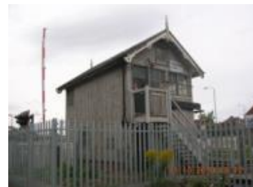
Figure 3.167: View of Signal Box from south east.
