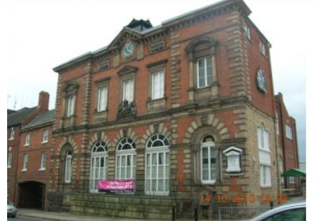
Figure 3.12: South elevation (original frontage) of Town Hall from 1970 and present day (source: Bassetlaw Museum, 2010).
