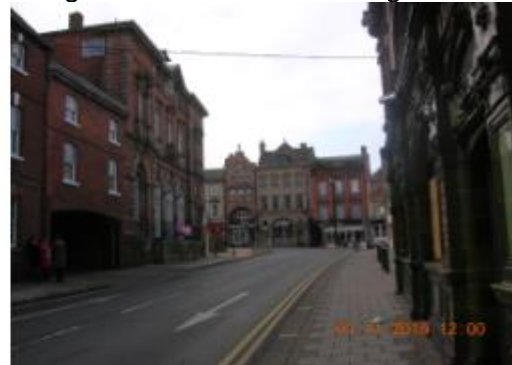
Figure 3.53: View westwards along Potter Street towards Bridge Street and Town Hall (left).
