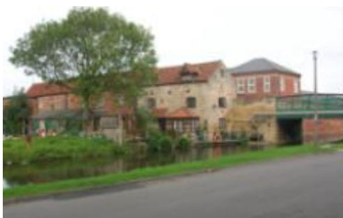
Figure 3.103: View of buildings to west (centre) and east (distant right) of Kilton Road, with canal bridge also shown (right).
