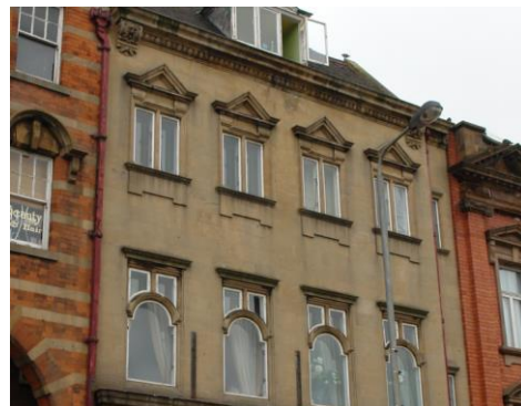
Figure 3.31: Windows at 116 Bridge Street.
