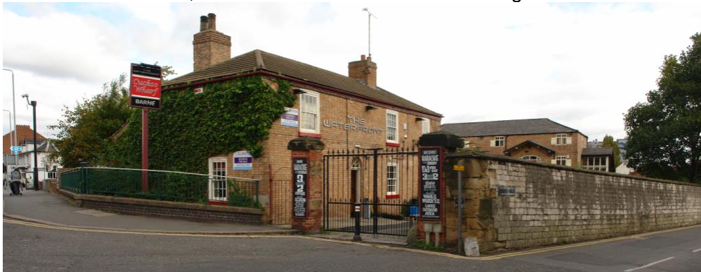
Figure 3.109: Former canal cottage, now Waterfront (public house), viewed from south west.
