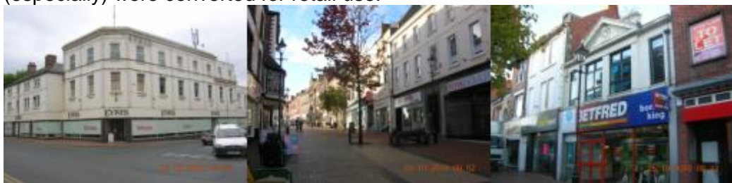
Figure 3.43: Left: Segmented window headers with large keystones at Eyres, Park Street; Centre: Squared architraves at 100-104 Bridge Street; Right: Pediment at 44 Bridge Street.
