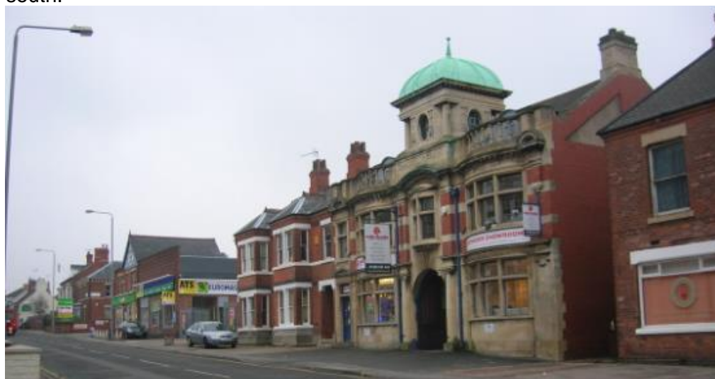
Figure 3.171: Former Council offices, viewed from south west.
