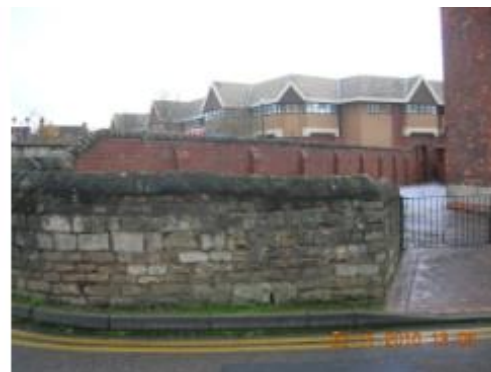
Figure 3.128: View of stone/brick wall to west of No.37 Church Walk.
