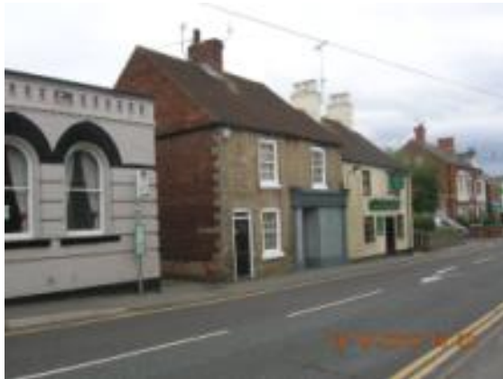
Figure 3.172: View of 90-92 Carlton Road, from north west.
