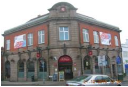
Figure 3.115: View of former Gas Showroom from North east.
