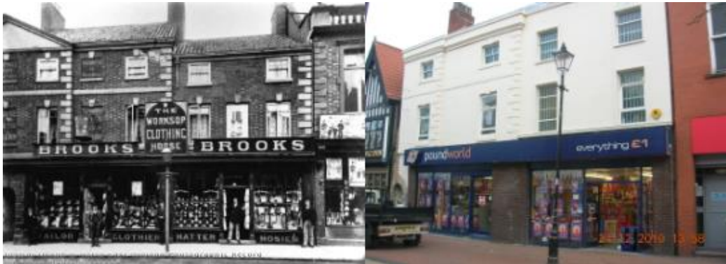
Figure 4.3: 39 & 41 Bridge Street, in 1900 (left) and present day (right). A significant number of unsympathetic changes appear to have been made to this building in the 20 th century, including the replacement of timber windows with UPVC, the bricking up of other windows and the replacement of the 19 th century shop fronts. The box signage is particularly intrusive, as it stretches the full width of the building and projects away from the building. Source: www.picturethepast.org.uk , 2010.
