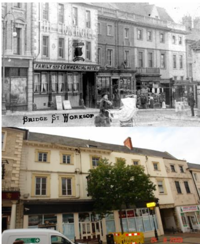
Figure 3.18: Frontage of 106, 108 & 110 Bridge Street from c.1890 and present day (source: Bassetlaw Museum, 2010).
