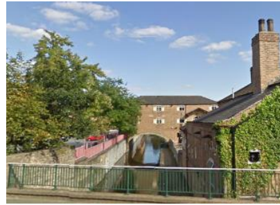
Figure 3.129: View of canal depository from bridge to west, looking east.
