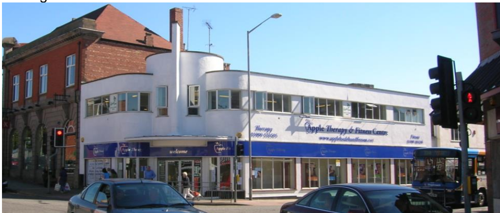
Figure 3.121: View of 7-9 Bridge Place, from south west.
