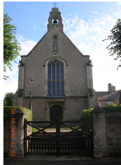
Figure 3.37: West elevation of St. Mary’s Roman Catholic Church, facing Park Street.
