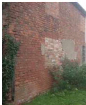
Figure 3.30: Chandos Court. Note the Georgian period Flemish brick bond and rubbed brick window arches (source: BDC, 2010).
