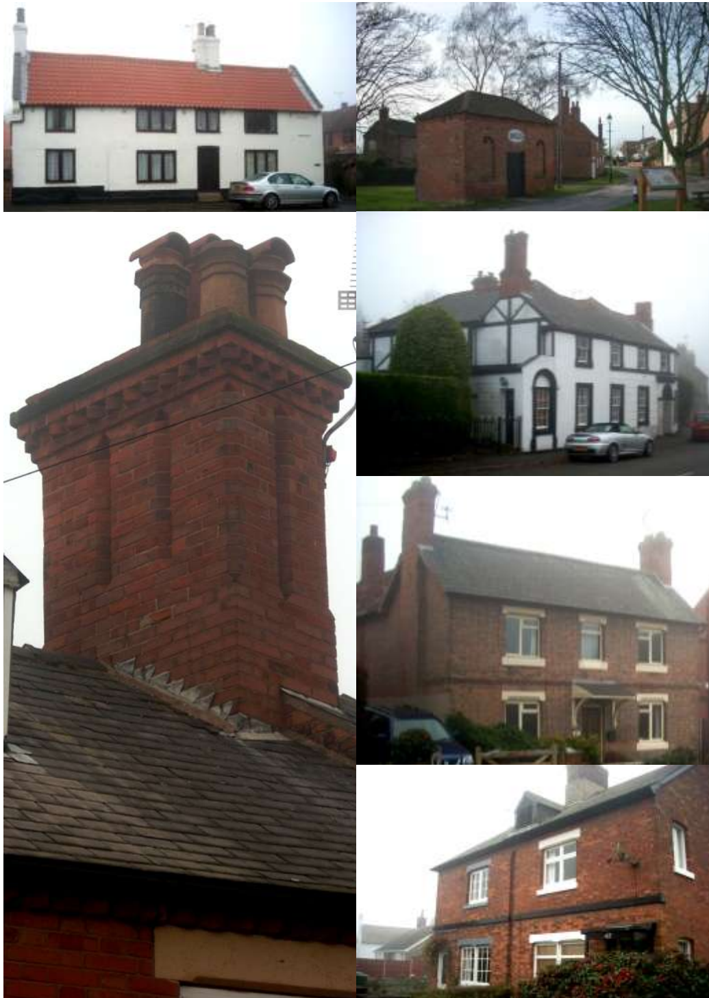
Figure 3.53: Roofs are a mixture of clay pantiles and slate on historic buildings. Houses have chimney stacks, predominantly with brick detailing such as oversailing courses (source: BDC, 2010).
