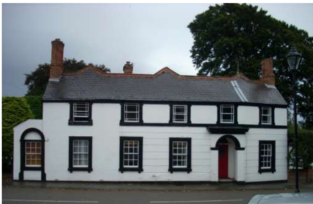
Figure 4.3: Historic timber windows and chimney stacks are an important feature of this building. The Conservation Area quality would be lessened if windows were replaced with UPVC or if chimney stacks were removed (source: BDC, 2008).
