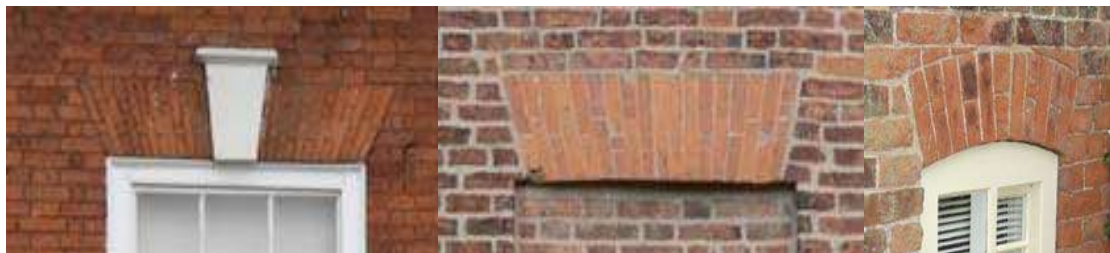
Typical window headers with both cambered and arched brick detailing.
