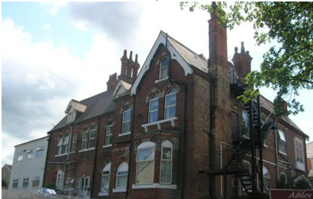
Figure 2.2: View of former Water Works manager's house, currently a nursing home.
