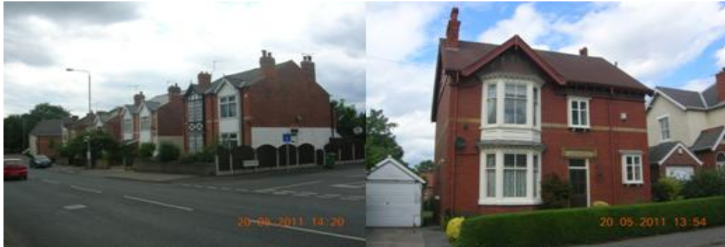
Figure 3.18: View of buildings in setting of Conservation Area, including early 1900s semi-detached houses on west side of Carlton Road (left) and 13 Beech Avenue (right).
