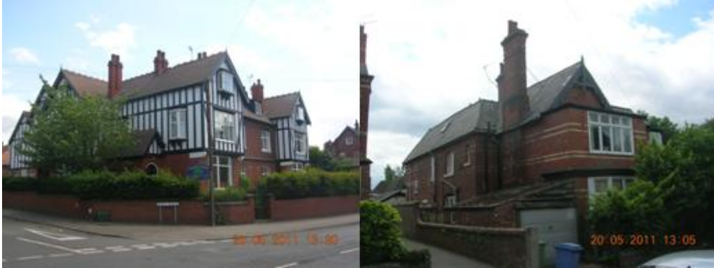
Figure 3.23: Walls and hedging at 292 & 294 Carlton Road (left); boundary wall with curved section between 4 and 2 Sunnyside (right).
