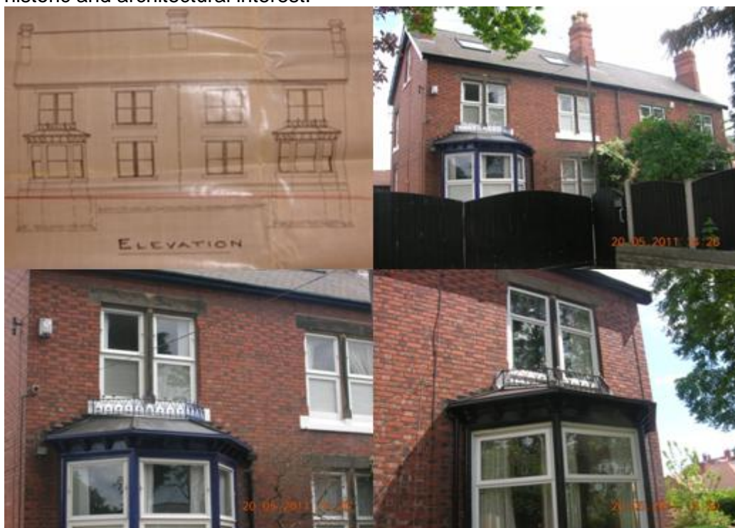
Figure 3.16: Frontage of 298 Carlton Road/1 Beech Avenue from original plan by Alfred Appleby & Son, 1902 (top left) and present day (top right); bay windows with decorative iron work at both properties (bottom left and right) and original metal-framed centre pivot windows at 298 Carlton Road (bottom left).
