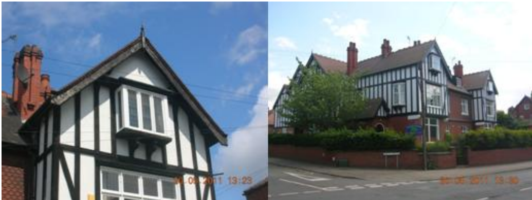
Figure 3.14: Original windows at 2 Sunnyside (left); 292 & 294 Carlton Road, as viewed from point on Carlton Road to north west (right).
