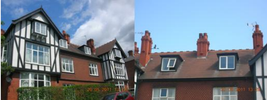
Figure 3.13: Frontage of 290 Carlton Road/2 Sunnyside (left); prominent chimney stacks at 292 & 294 Carlton Road (right).
