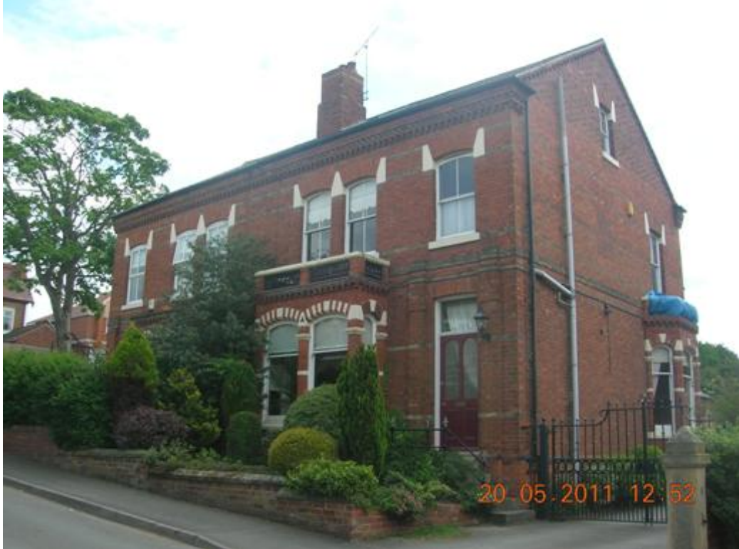
Figure 4.2: Here the window bays, sliding sash windows and central chimney stack are important features on this building and in the wider setting. The character of the Conservation Area would be detrimentally affected if bays were removed, UPVC windows were installed or if the central chimney stack was removed.
