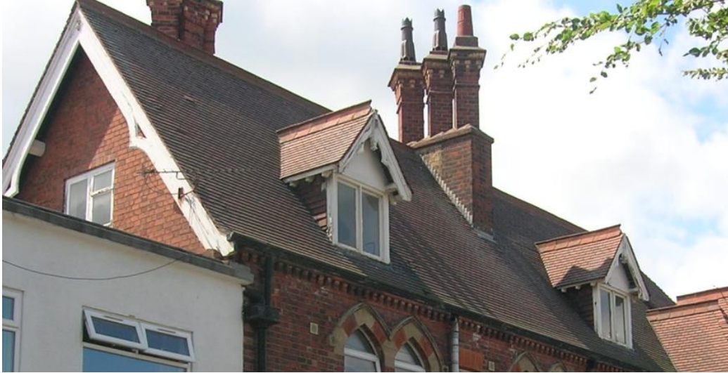
Figure 3.4: View of highly decorated chimney stacks, dentil coursing, arched window headers and dormer windows with bargeboards, from north east.
