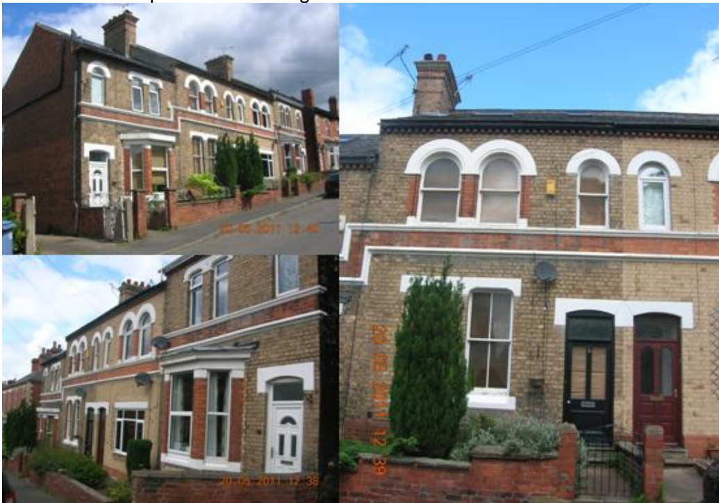
Figure 3.9: Views of frontage of 7-13 Sunnyside from south west (top left) and from south east (bottom left); frontage of 9 Sunnyside, featuring original timber sash windows and door (right).
