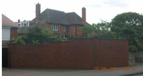
Figure 3.17: 280 Carlton Road, viewed from point on Carlton Road from north west.
