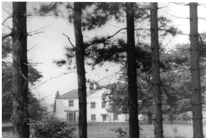
Scaftworth Hall, a Grade II listed building (source: BDC, 2010).
