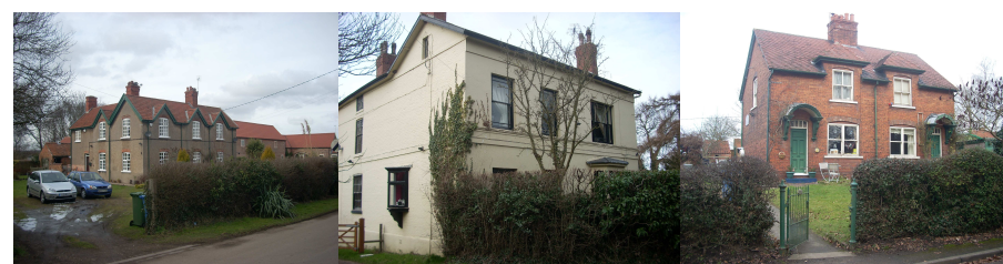
Scaftworth has a coherent architectural form (source: BDC, 2010).
