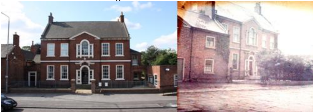
Figure 3.74: Frontage of Amcott House, including historic image showing original railings (right). Image source: Bassetlaw Museum, 2011.
