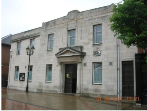
Figure 3.109: Frontage of Court House, Exchange Street.
