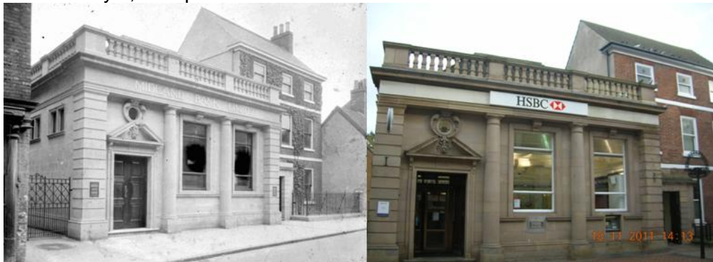
Figure 3.108: Former London Joint City & Midland Bank, Carolgate, from 1925 (left) and present day (right). Image source: Bassetlaw Museum, 2011.
