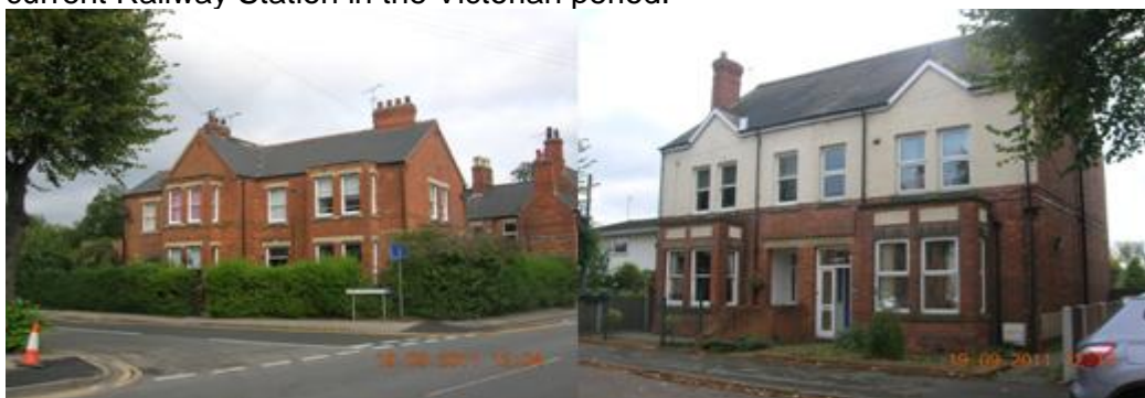
Figure 3.40: Buildings on Lime Tree Avenue: Number 2 (left) and 21-23 (right).
