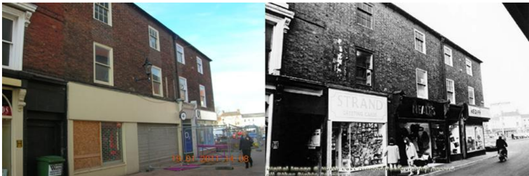
Figure 4.5: The replacement of the 19 th century shop fronts (visible on the 1960 photograph, right) has resulted in an incongruous feature on this historic building range. Image source: www.picturethepast.org.uk , 2012.
