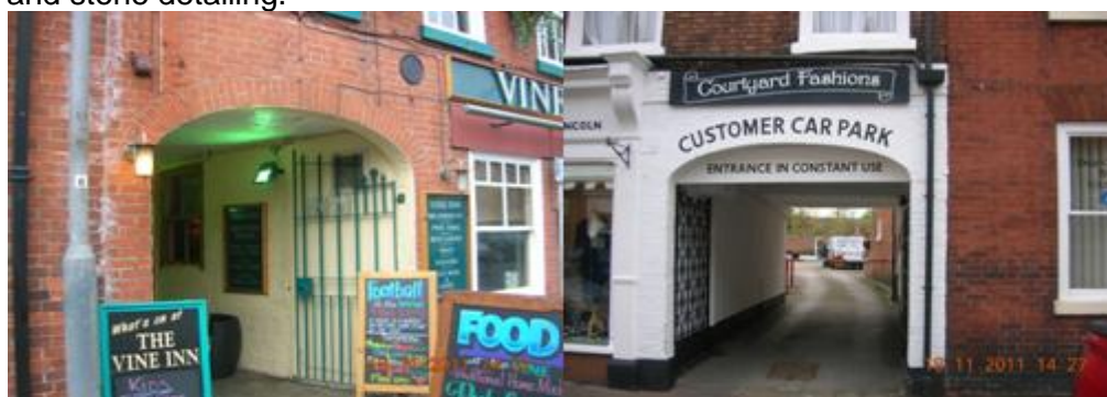
Figure 3.80: Coach accesses with brick arches at Churchgate (left) and Grove Street (Right).
