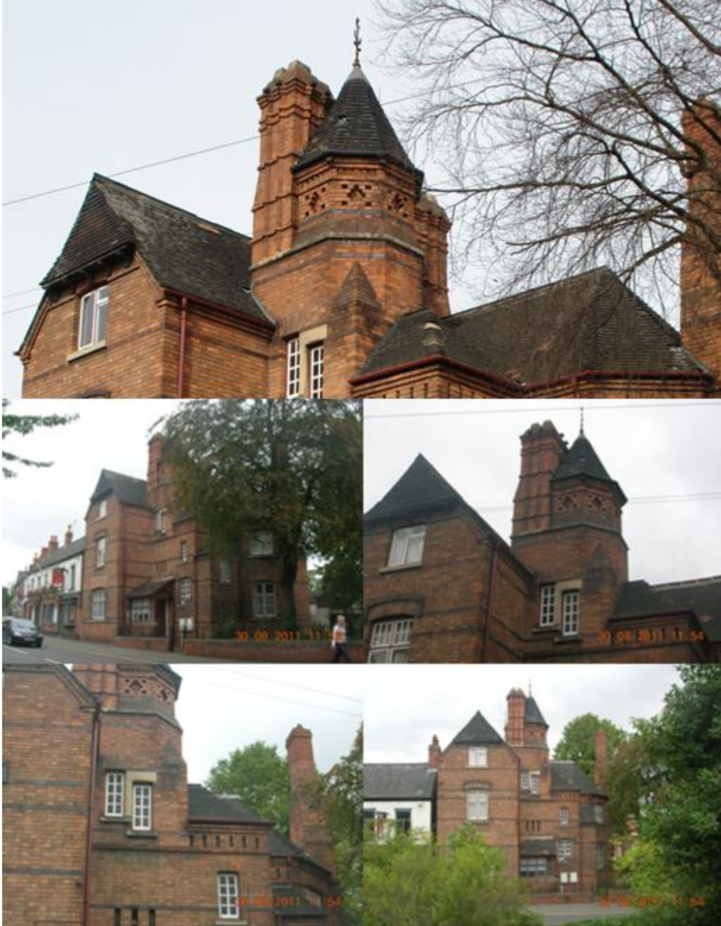
Figure 3.28: Further views of Sandrock House (60 Bridgegate), including geometric brickwork pattern on turret.
