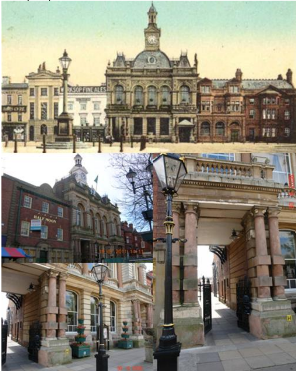
Figure 3.95: Views of Town Hall frontage, including image from c1900 (top) and columns/balconies (bottom left and right). Image source: www.picturethepast.org.uk , 2011.
