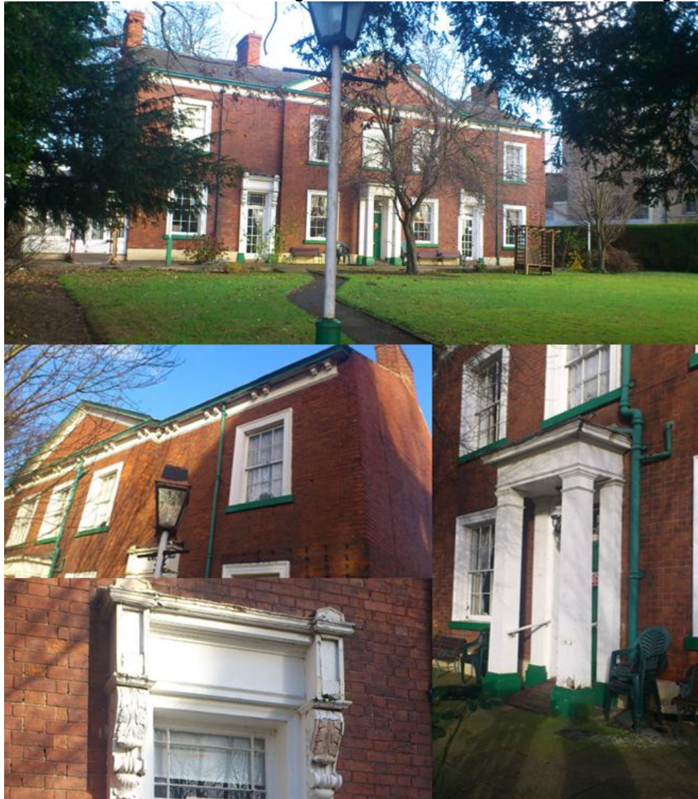
Figure 3.167: Frontage of The Hollies, showing eaves detailing and windows (top and centre left), central doorway (bottom right) and side doorway with foliated mouldings (bottom left).
