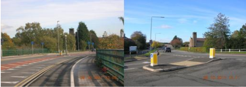
Figure 3.61: Views of the Catholic Church from Babworth Road, from west (left) and east (right).
