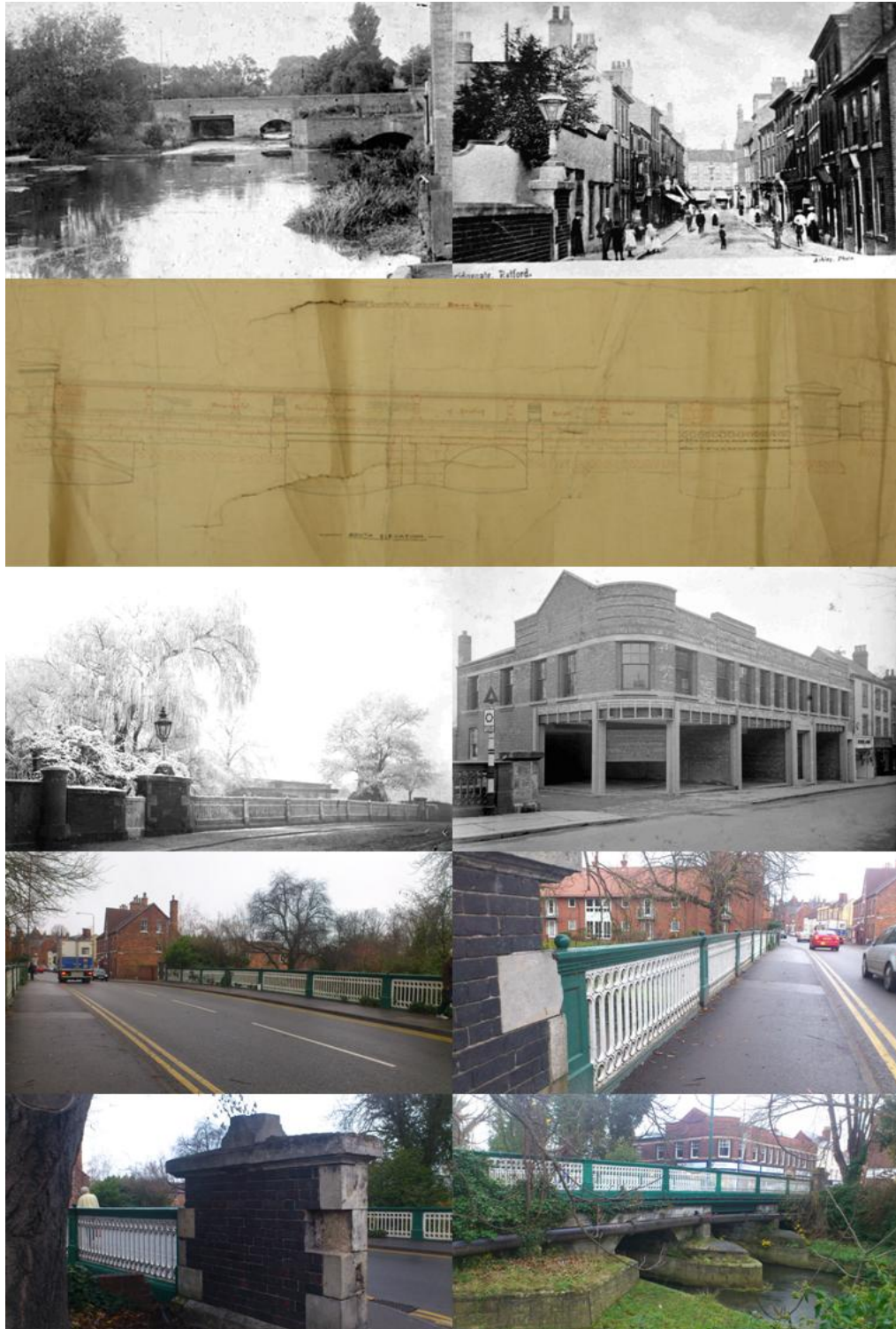
Figure 3.125: Top row: Bridgegate Bridge, as shown in c1900 with original brickwork and gas lamps; Second row: later iron balustrading in alteration plan from early 20 th century; Third row: photographs of bridge from c1900-1910 (left) and 1937 (right); Elsewhere: Bridgegate Bridge, present day.
