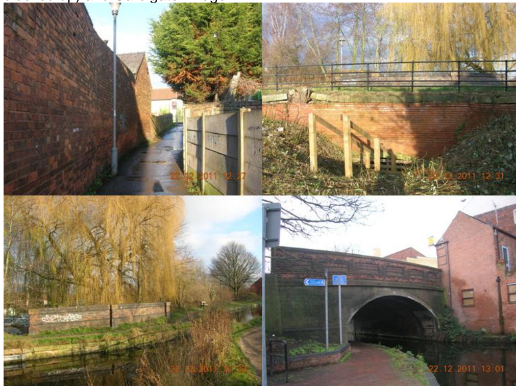
Figure 3.155: 19 th century brick boundary wall to south of Chesterfield Canal (top left), late-18 th century brick and limestone underpass structure (top right), early-20 th century wall above late-18 th century aqueduct (bottom left) and early-20 th additions to Carolgate Bridge (bottom right).
