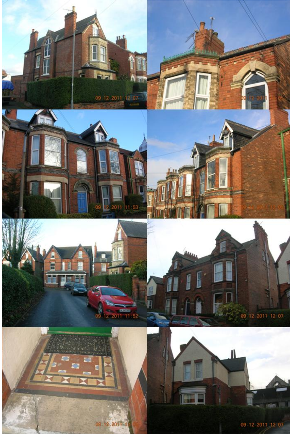
Figure 3.178: Various late-19 th /early-20 th century houses on Holly Road.
