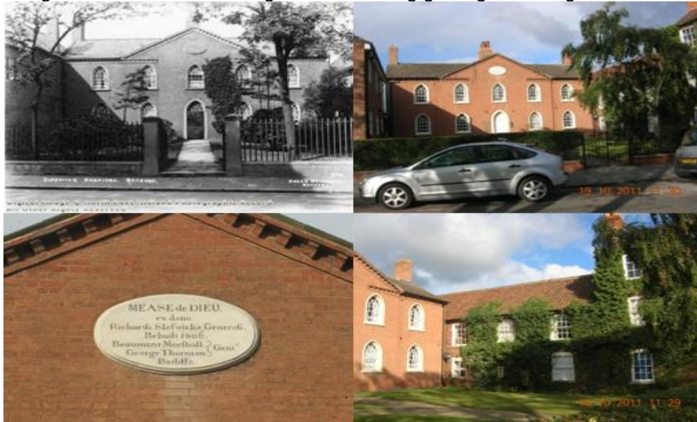
Figure 3.82: Views of Sloswick's Hospital Almshouses, including from c1920 (top left) and feature tympanum plaque within pediment (bottom left).
