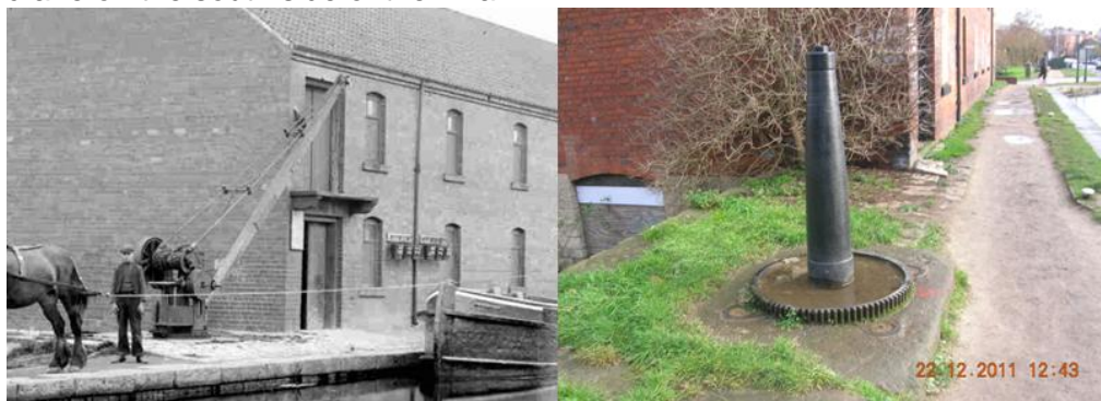
Figure 3.141: Original crane structure in c1900 (left) and surviving central shaft (right). Image source: www.picturethepast.org.uk , 2011.
