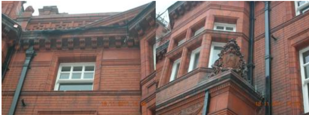
Figure 3.105: Decorative dentil coursing and cast iron rainwater goods (left) and million/transom windows and coat of arms (right) and former Foljambe's Bank, The Square.
