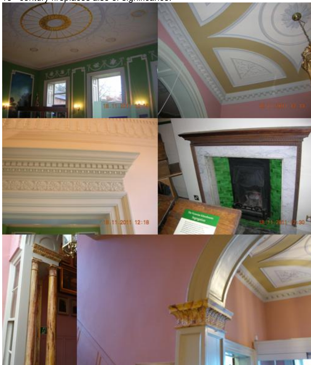
Figure 3.75: Internal features at Amcott House, including intricate plaster ceilings (top), door architrave (centre left), 19 th century fireplace (centre right), marble columns supporting Palladian opening (bottom left) and moulded columns with marble capitals (bottom right).
