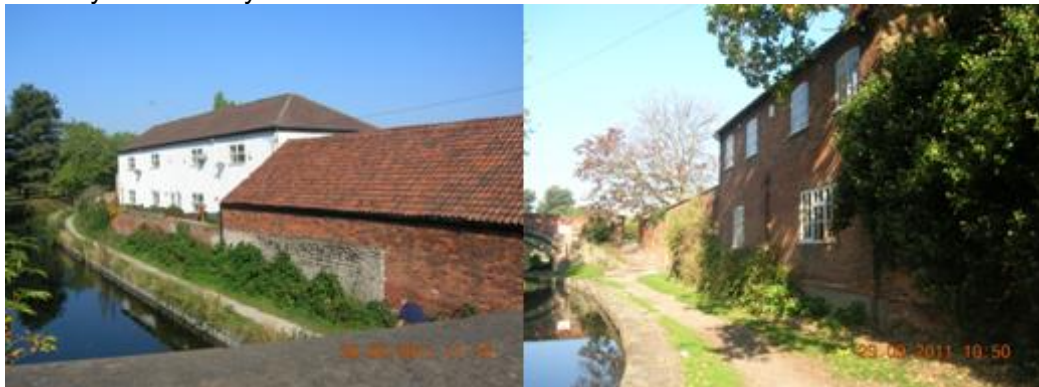
Figure 3.18: Buildings alongside Chesterfield Canal, with former maltings at Hannam's Yard (left) and Abberley (right).
