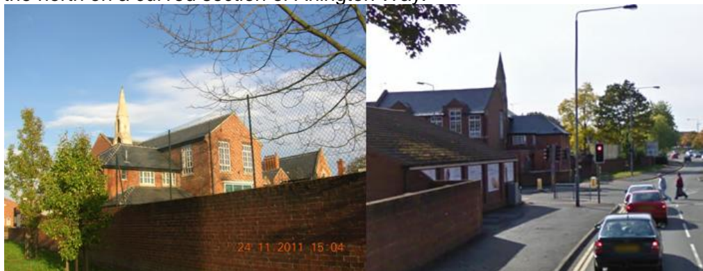
Figure 3.133: Bellcote at St Swithun's School, as viewed from points along Arlington Way to south west (left) and north (right).
