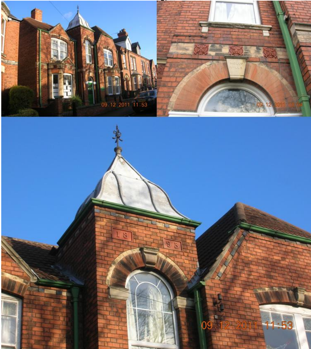
Figure 3.179: Views of Holly Villa, including leaded pinnacle and terracotta date tiles (top right), window arch detailing (bottom left) and original front door (bottom right).
