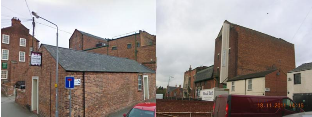
Figure 3.134: Views of Majestic Theatre fly tower from Exchange Street (left) and from Coronation Street (right). Image source: Google Maps, 2011.
