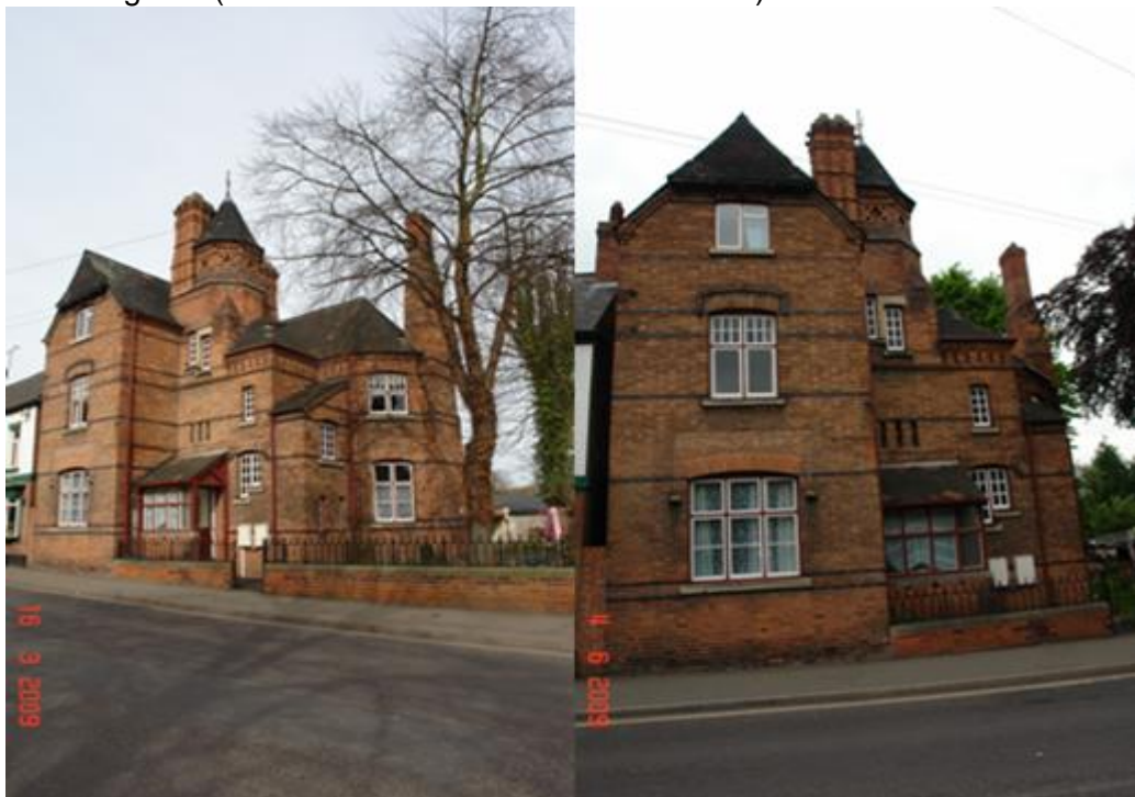
Figure 3.27: Sandrock House (60 Bridgegate), by Watson Fothergill, 1877, as viewed from Bridgegate.
