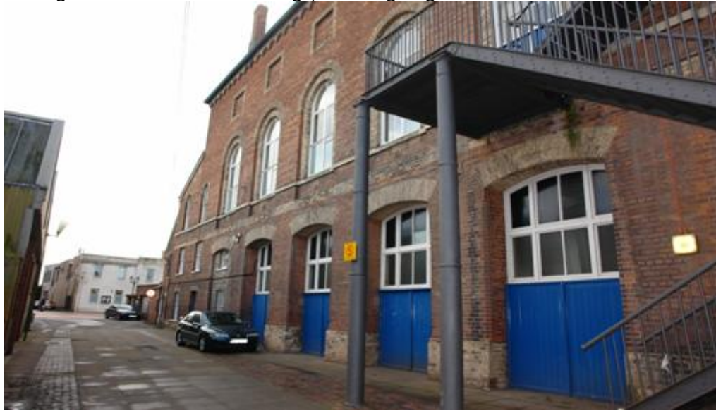
Figure 3.96: View of rear of Town Hall building (Butter Market).
