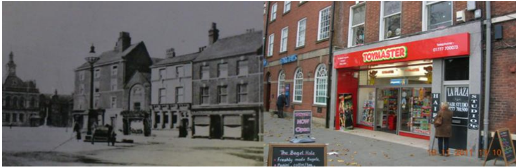
Figure 4.2: The present shop front surround (grey tiles) was installed in the 1950s, replacing the mid-19 th century timber shop front shown on the 1890 photograph (left). Image source: Retford Library, 2012.
