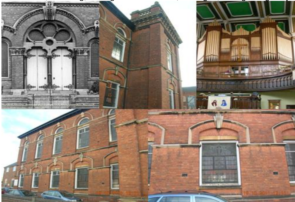
Figure 3.92: Views of Wesleyan Methodist Church building, including double entrance with original timber doors (replaced with glass in 1995) from c1970 (top left), internal view showing organ, gallery and decorated roof (top right), western frontage tower as viewed from Union Street (top centre) and windows facing Union Street (bottom). Image source: Bassetlaw Museum, 2011.
