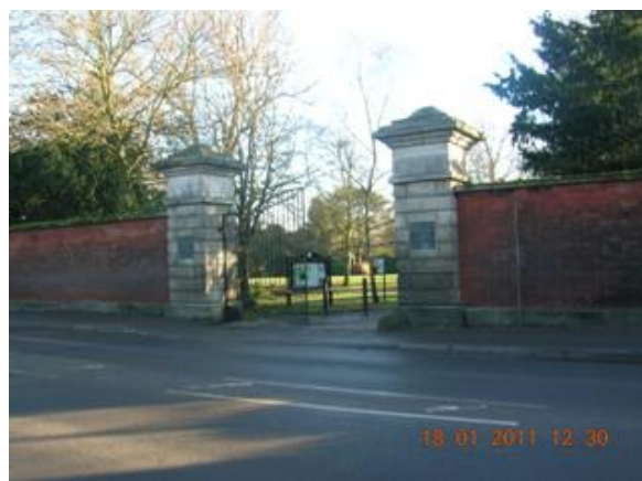
Figure 3.56: Hospital Road: Brick wall around Kings' Park, with early-20 th century inserted gateway.
