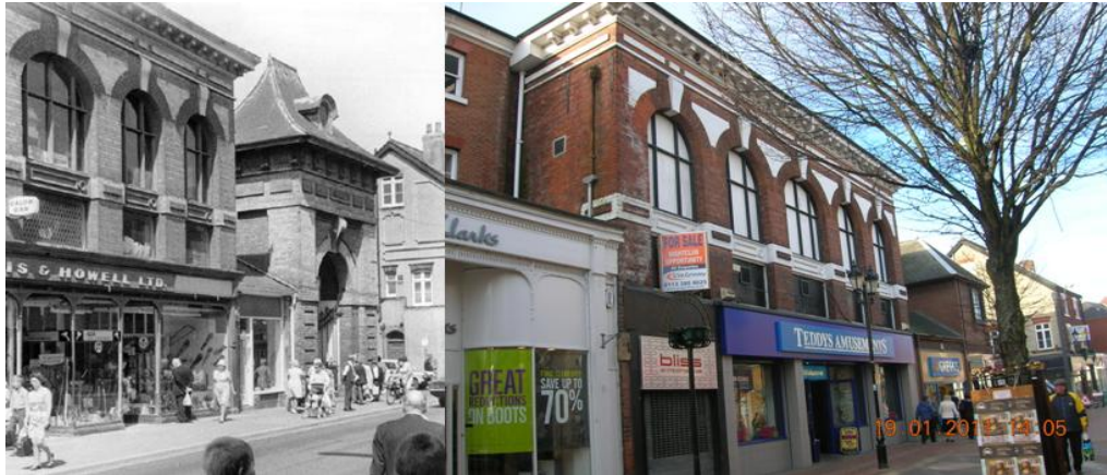
Figure 3.107: Views of frontage of 20 Carolgate from 1971 (left) and present day (right). The early-20 th century iron and glass shopfront is clearly visible on the 1971 picture. Image source: www.picturethepast.org.uk , 2011.
