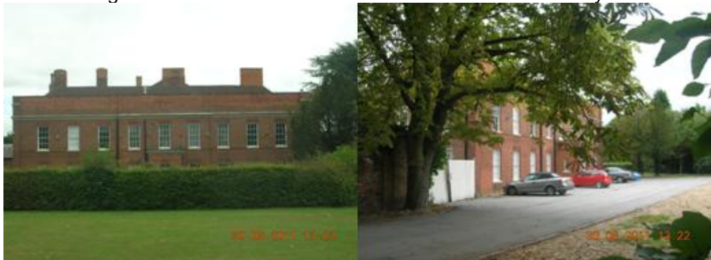
Figure 3.6: Views of main frontage (west elevation) of West Retford Hall.
