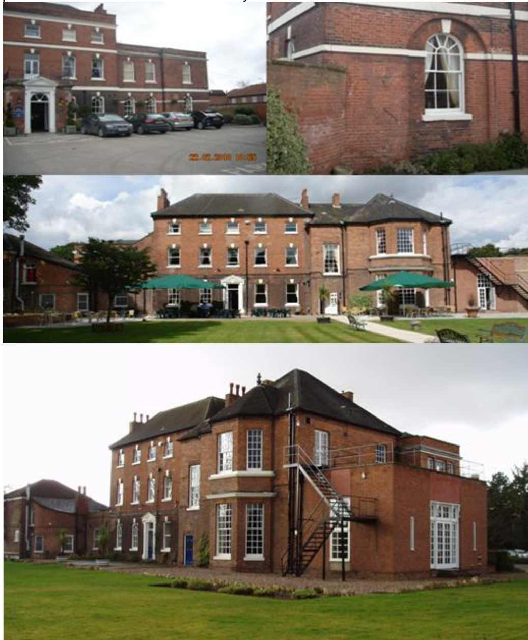
Figure 3.12: Views of West Retford House, including right hand bay of frontage (top left), original half-round niche (top right) and rear aspect (centre and bottom).
