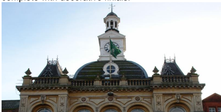
Figure 3.94: Frontage roof of Retford Town Hall
