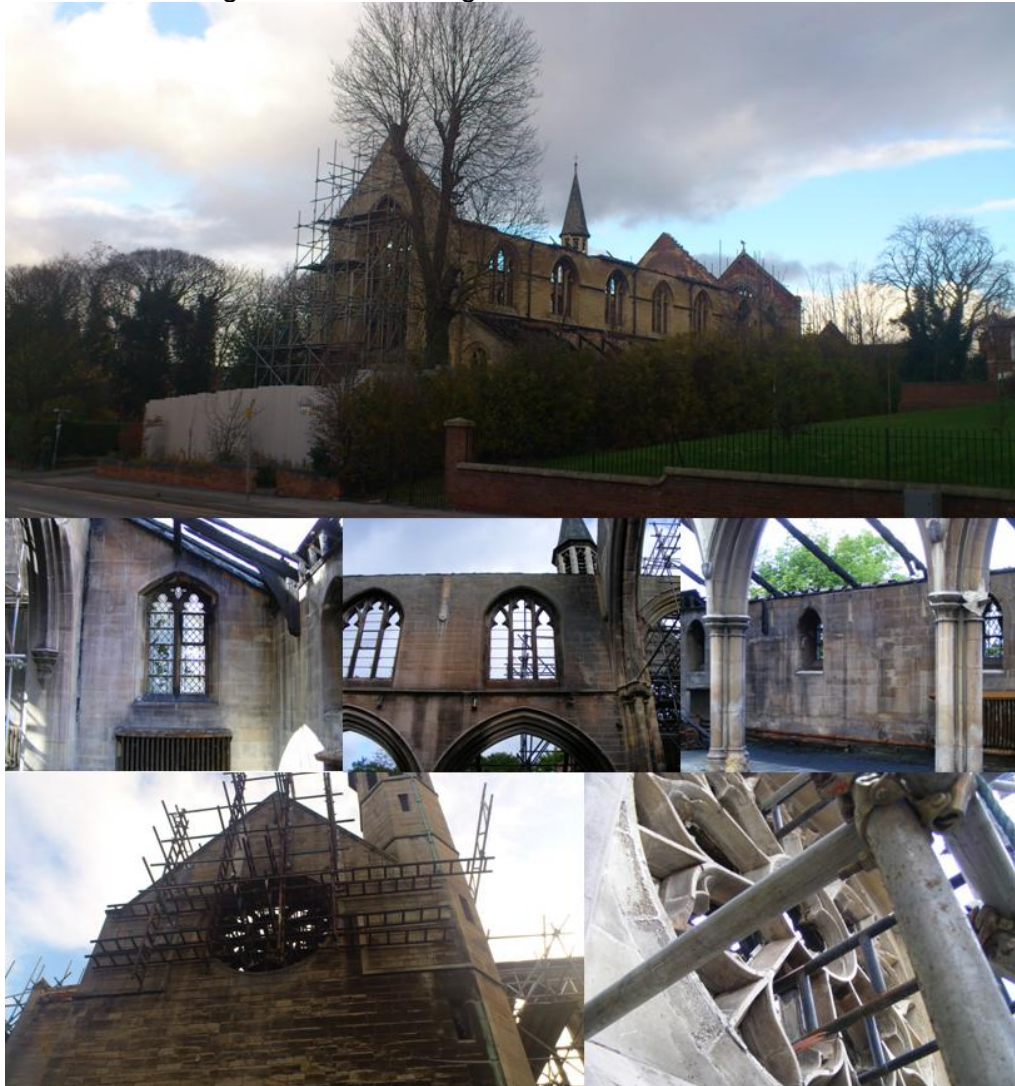
Figure 3.174: Views of St Alban's Church, from London Road (top), from inside (centre) and of circular window opening with tracery on north side (bottom).
