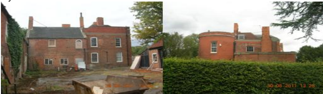
Figure 3.8: Views of West Retford Hall, showing north elevation (left) and south elevation complete with rounded bay on the south east corner (right).
