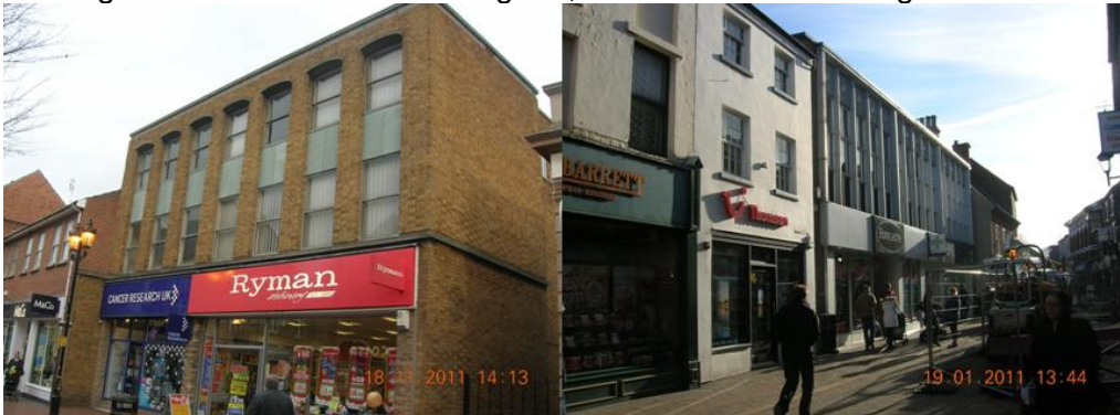
Figure 3.116: Modernist architecture of 27 Carolgate (left) and 11-15 Carolgate (right).
