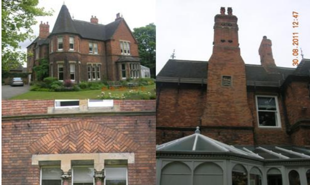
Figure 3.22: Views of former West Retford Rectory (by James Fowler, 1864), including turret at south west corner (top left), decorated chimney (right) on east elevation (main frontage) and brick arch with herringbone-pattern brickwork (bottom left) on south elevation.
