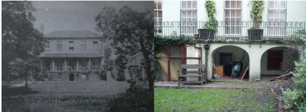
Figure 3.164: Rear of Ordsall House, from c1900 (left) and present day (right). Image source: Retford Library, 2011.
