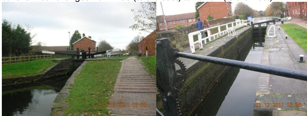
Figure 3.138: East Retford Town Lock, showing limestone (left) and engineering brick (right).
