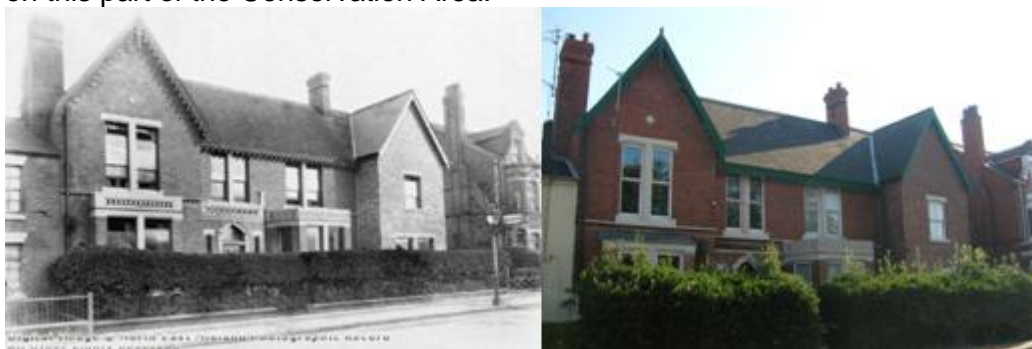
Figure 3.33: Lorne House, Queen Street, as seen in 1926 (left) and present day (right). Image source: www.picturethepast.org.uk , 2011.
