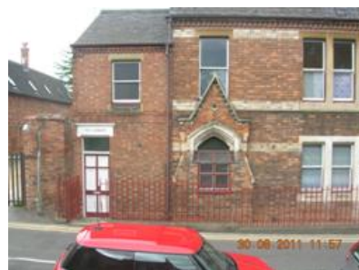
Figure 3.30: Gothic-style arch at Darrel House, Rectory Road.
