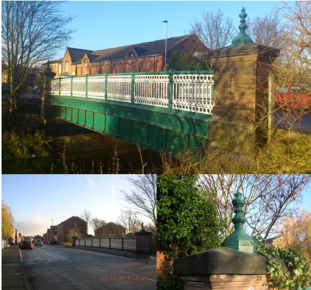
Figure 3.160: Albert Road bridge, as viewed from south east (top) and west (bottom left). Also shown is one of the four lamp bases (bottom left).
