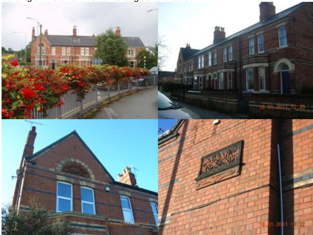
Figure 3.38: Views of 1-7 North Road, including frontage (top and bottom left), decorative half-round panel (bottom left) and feature date panel on side (bottom left).
