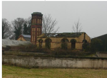
Figure 2.9: Former Pumping Station, Bolham Lane.
