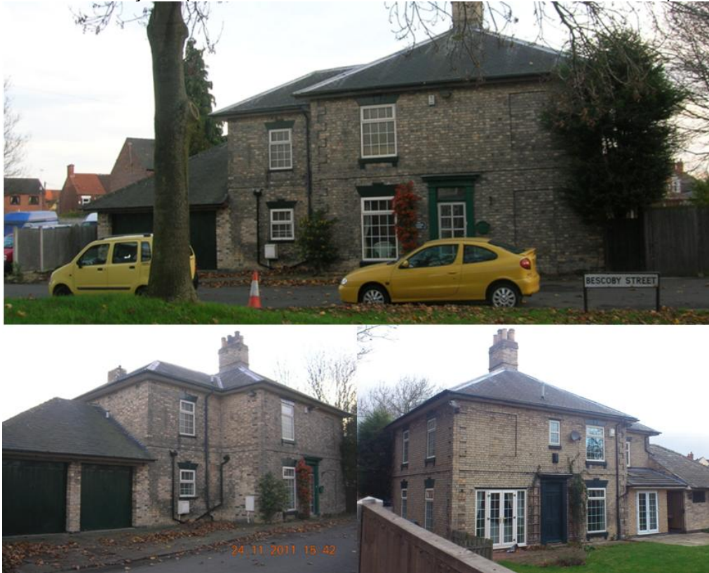
Figure 3.101: Views of Spa Common House, from Spa Common/Bescoby Street (top and bottom left) and from Chesterfield Canal (bottom right). Tax relief openings are clearly visible.
