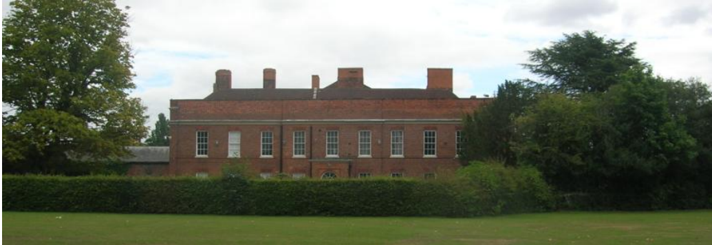
Figure 3.7: Main frontage of West Retford Hall.
