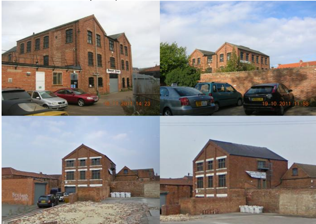
Figure 3.111: Industrial buildings between Carolgate and Beardsalls Row (top) and between Carolgate and Canal Street (bottom).
