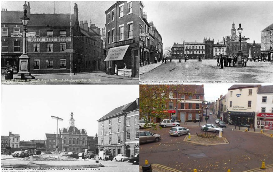
Figure 4.6: The junction of Market Square and Bridgegate currently has damaged surfacing, unsympathetic highway interventions and a small brick roundabout structure. Within this structure, a traditional-style triple lamp structure exists, although has modern plastic planters on the supporting column. Whilst this is an improvement on the large 1960s roundabout (bottom left), during the Victorian period this area contained a large feature gas lamp (see 1900 photographs, top) which also had directional signs on the column. Image source: www.picturethepast.org.uk , 2011.
