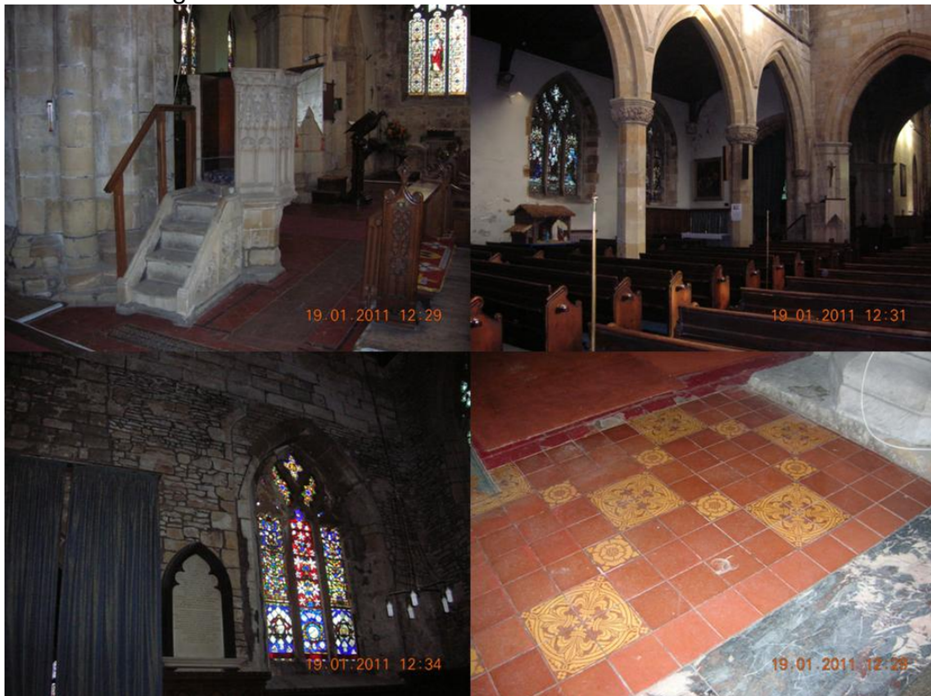
Figure 3.66: Views of north transept and tower arch at St Swithun's, including Late-Medieval column with 19 th century support (top), comparison between Medieval and Victorian masonry on inside wall (bottom right) and mid-19 th century floor tiles around earlier column (bottom right).
