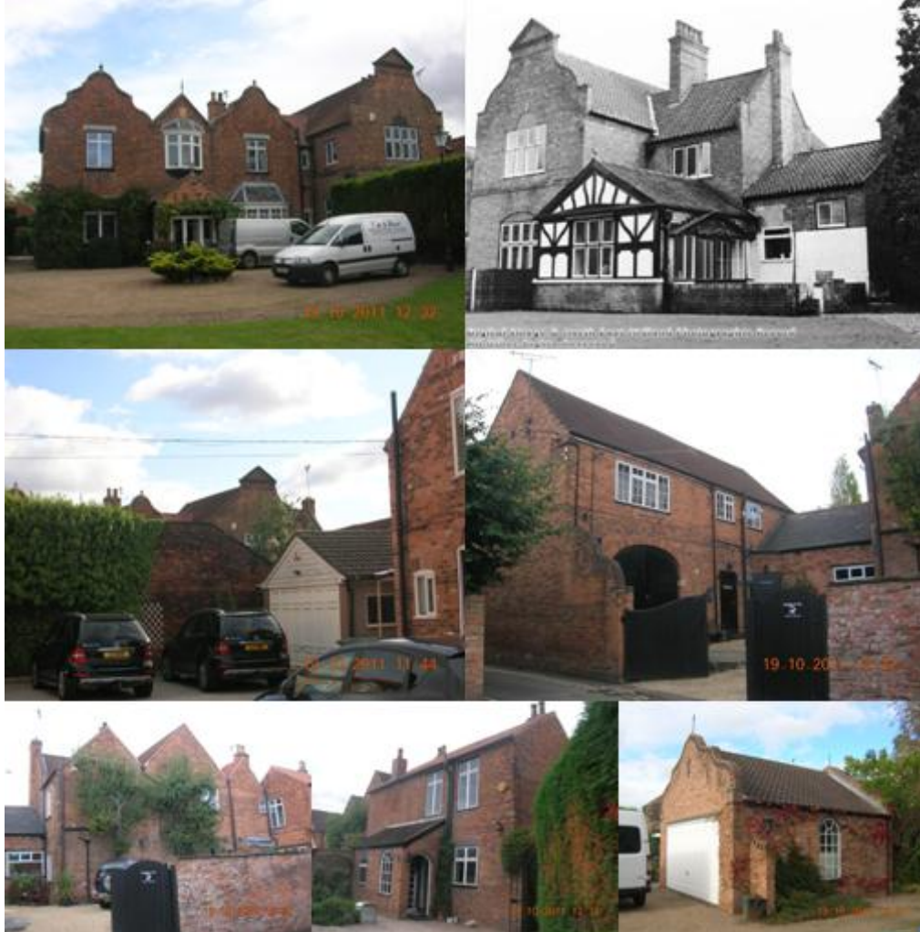
Figure 3.100: The Cloisters (top left) and Friar's Court (top right, from 1970), with their decorative Flemish gables, also visible from adjacent public car park (centre left). Less decorative frontages (bottom left and centre), former coach house (centre right) and modern buildings in same style (bottom right).
