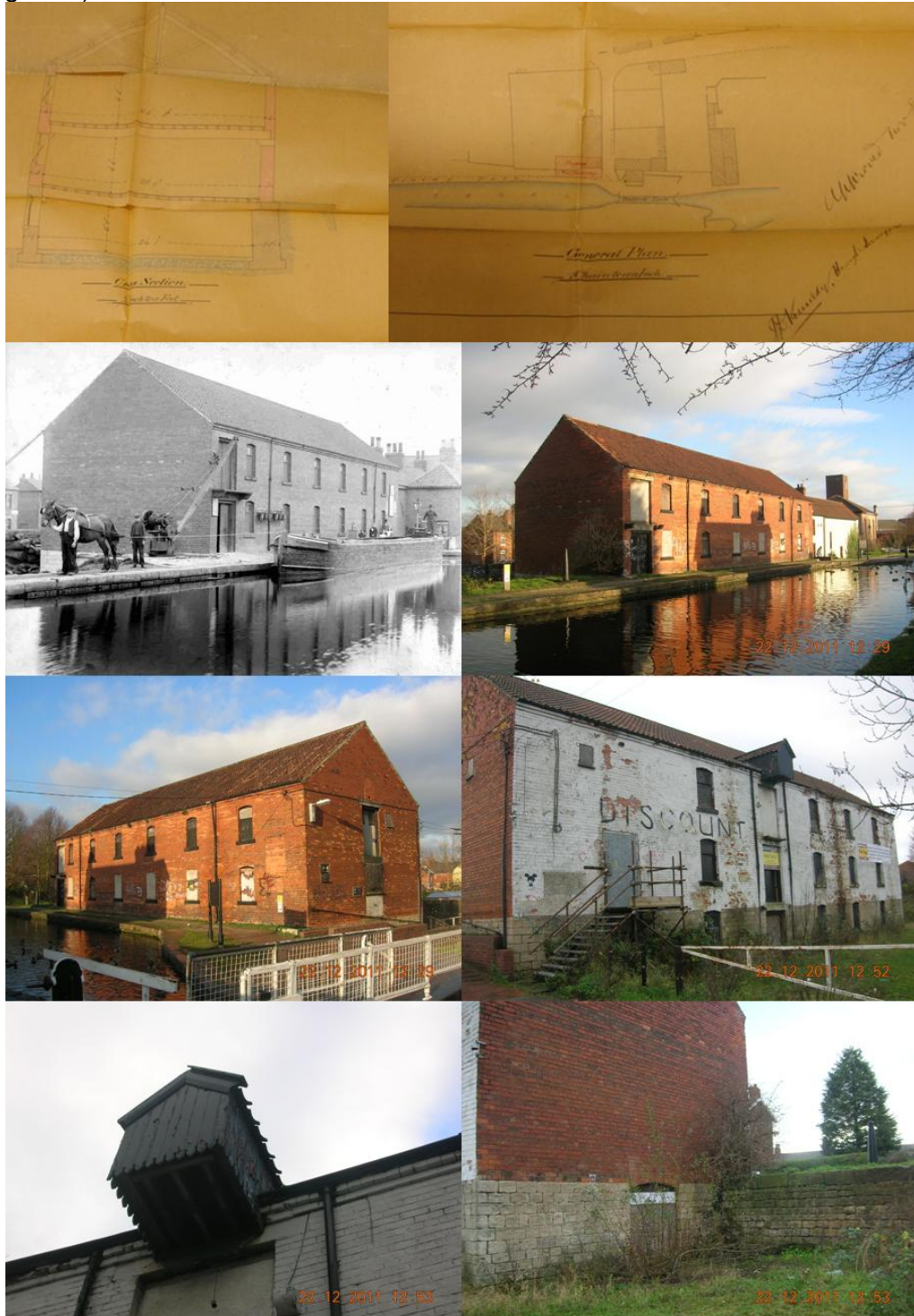
Figure 3.140: Former MSLR Warehouse, including original 1882 plan (top), image from c1900 (second row, left) and pulley wheel housing (bottom left). Plan source: Bassetlaw Museum, 2011. Image source: www.picturethepast.org.uk , 2011.
