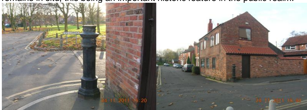
Figure 3.118: 19 th century sewer vent pipe at corner of Spa Common and Kirke Street.
