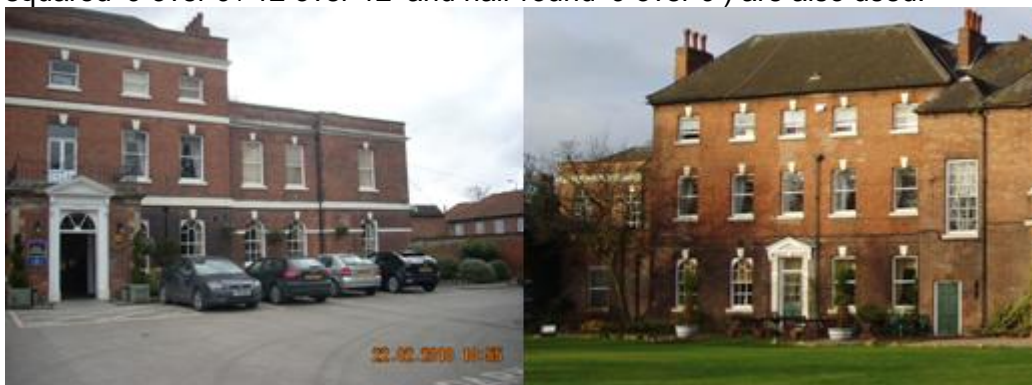
Figure 3.13: Different window types on front (left) and rear (right) of main building.
