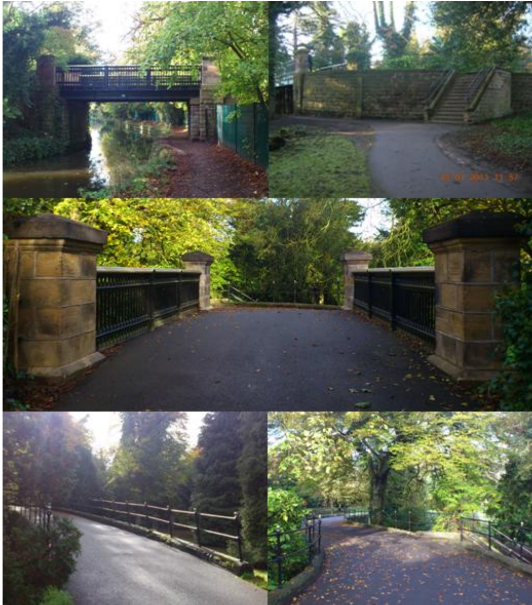
Figure 3.50: Views of Chesterfield Canal Bridge 54B, with its stone ramp/steps and iron balustrade/railings. The bridge connects the western and eastern parts of the cemetery.
