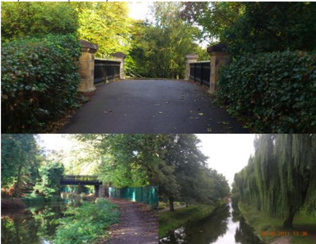
Figure 3.62: Views of Chesterfield Canal Bridge 54B from south (top) and south east (bottom left); view along River Idle, looking southwards from pedestrian footbridge (bottom right).
