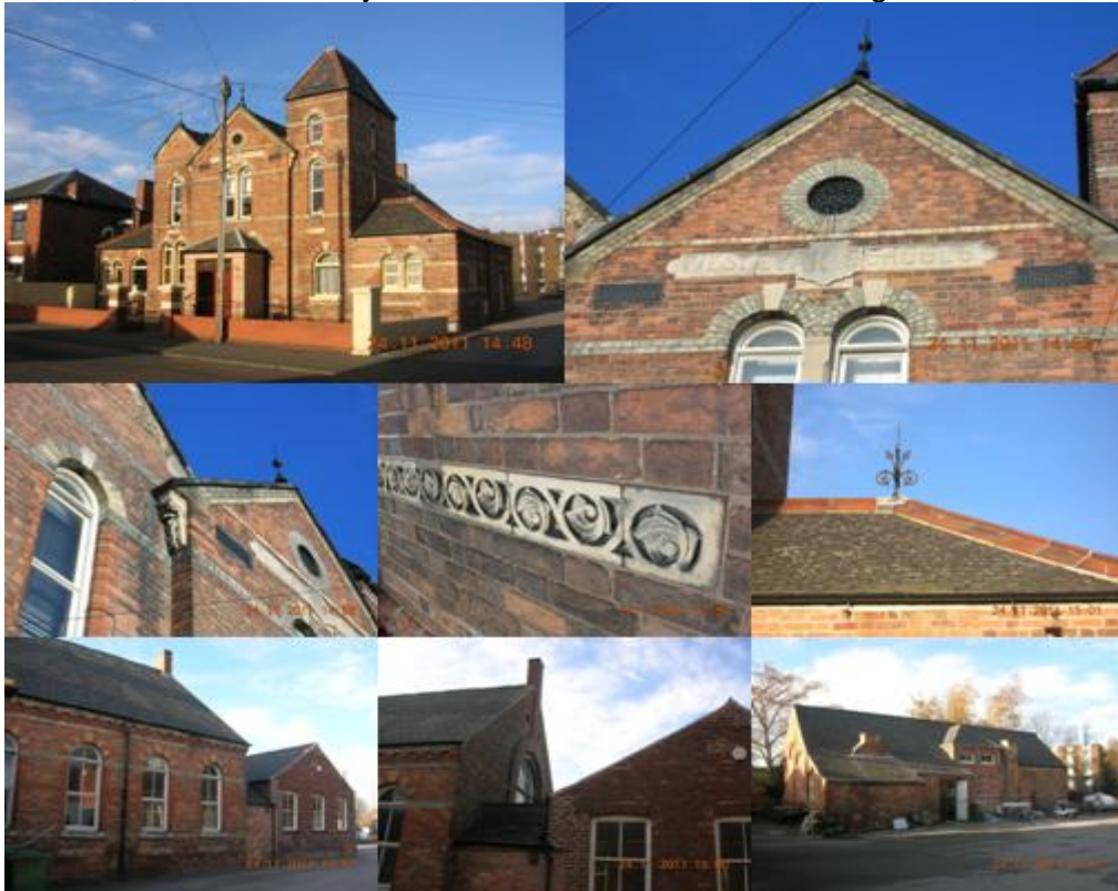
Figure 3.87: Views of former Wesleyan School, Grove Street, including frontage (top left), side/east elevation (bottom left) and former Wesleyan Infants' school to rear (bottom right). Decorative features include several finials (top right and centre right), moulded stone kneelers (centre left), carved stone panels (centre) and rear window on original building (bottom centre).
