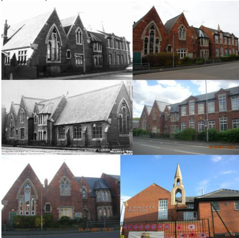
Figure 3.86: Replacement National School buildings on south side of Grove Street, including Infants' school (top), boys' school and former master's house (centre) and original and current girls' school (bottom). Image source: www.picturethepast.org.uk , 2011.
