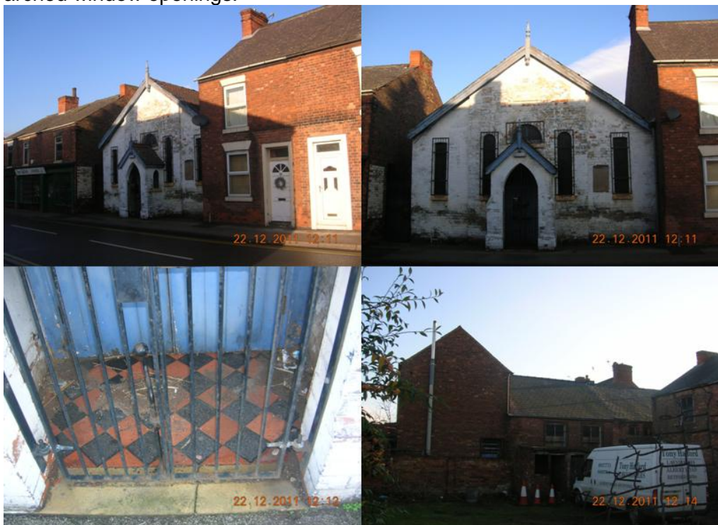
Figure 3.147: Views of former Albert Road Mission Hall, including of frontage (top), porch floor (bottom left) and side/rear (bottom right).
