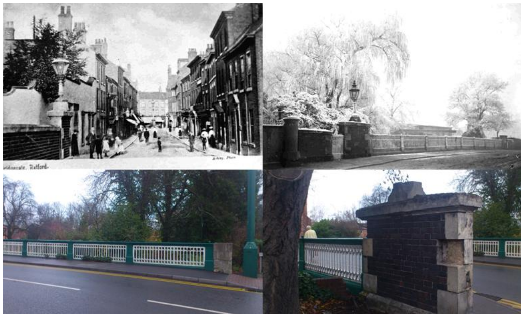
Figure 4.7: Bridgegate Bridge originally contained gas lamps (of the standard Retford Gas Works variety) at each of the four corners (see c1900 and c1910 photos, top left and right). The reinstatement of traditional-style lamps here would add greatly to the appearance of the bridge and the character of the wider streetscene. Image source: Bassetlaw Museum, 2011.
