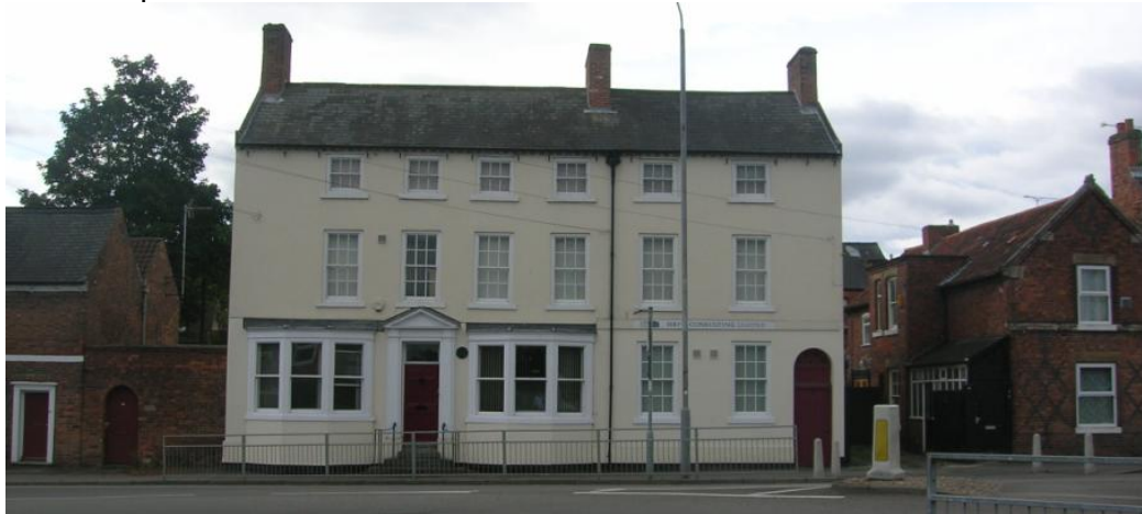
Figure 3.17: Frontage of 43 Bridgegate.
