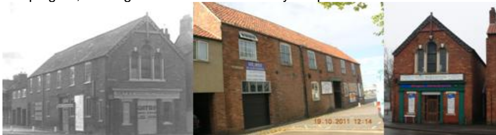
Figure 3.84: Former National School on corner of Chapelgate and Union Street.
