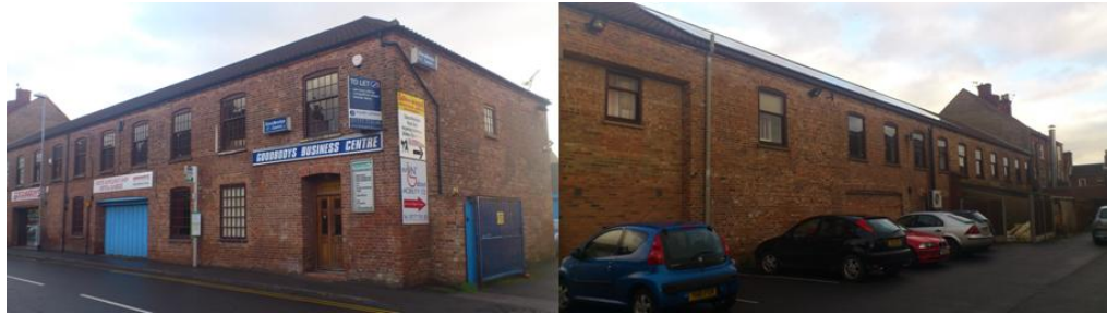
Figure 3.146: Frontage (left) and rear (right) of Goodbody's Mill building.
