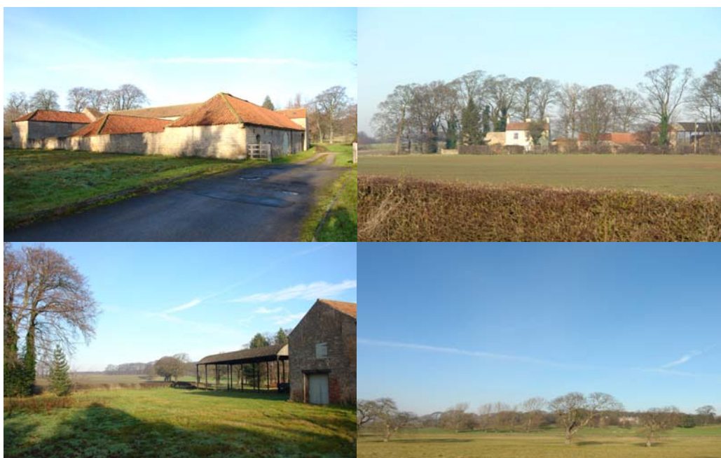
Figure 3.1: top left, the range of agricultural buildings at Gateford Hall possesses a characterful plan form; the adjacent farm range at California Farm (top right) is typical of a close-knit farm range; Gateford Hill character area layout (bottom left and right) is defined by agricultural buildings, field enclosures and the historic parkland of Gateford Hill House (source: Bassetlaw District Council, 2009).
