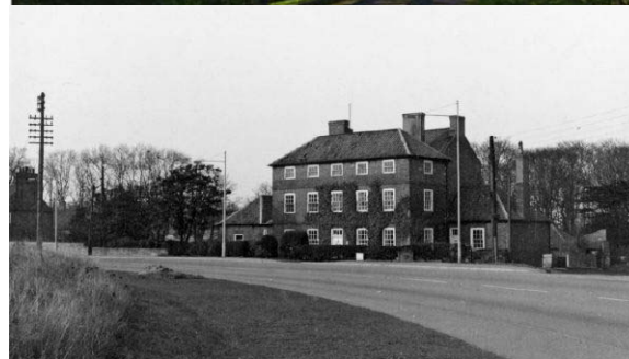
Figure 3.9: Gateford House. Top: the rear aspect of the house is the older part of the house (source: Bassetlaw District Council, 2008). Bottom: front view of the house from the 1960s (source: North East Midland Photographic Record, 2009).
