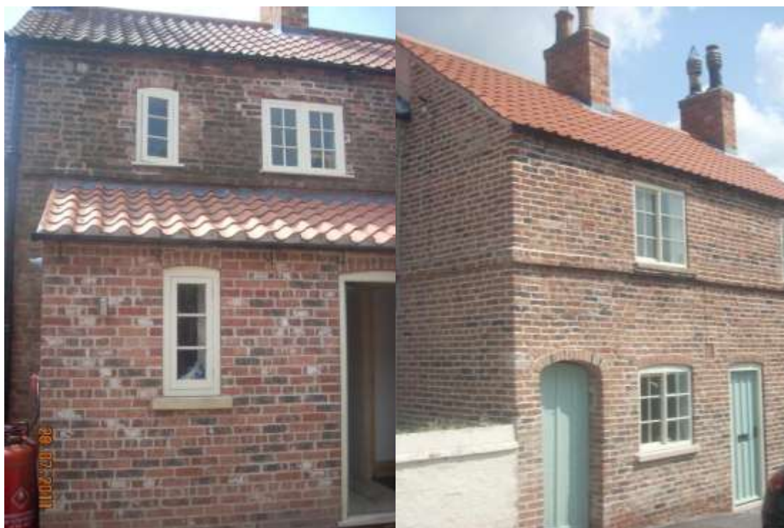
Left: A rear extension to an early 19 th century cottage has been constructed in modern block work, but has replicated English Garden Wall brick bond and brick arch headers, as well as using lime mortar in a flush/slightly recessed pointing finish. Right: Front of the cottage with traditional brick detailing, including string course, brick arches, flush verges and chimney stacks with oversailing courses.
