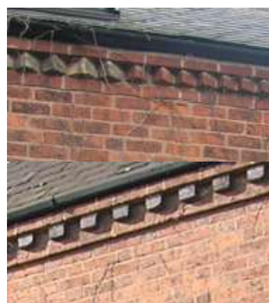
Dentil brick detail. Dog tooth (top) and simple projecting headers (bottom).
