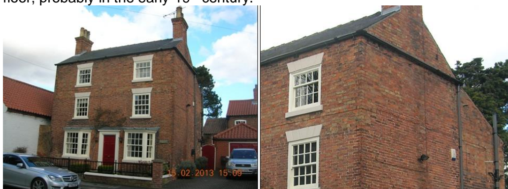
Figure 3.48: Views of Wood-Dene House, Church Street, with image on right showing change in brickwork demarking upper storey addition.
