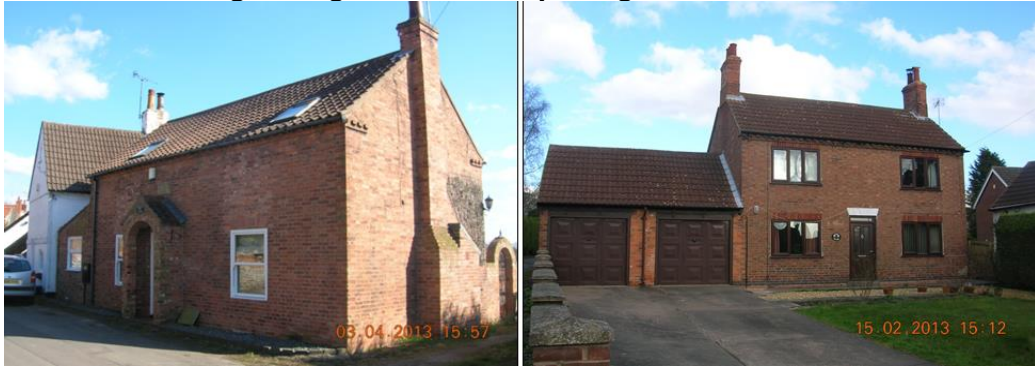
Figure 4.5: Loss of original window openings on Low Street (left) and enlargement of original openings on Church Street (right).
