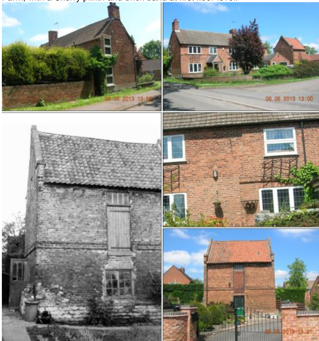
Figure 3.36: Bowerhayes as viewed from Plantation Road (top), showing distinct phases of brickwork including projecting brick band on south side (centre right) and listed dovecote with stone plinth in 1981 (bottom left) and present day (bottom right). Image source: Bassetlaw Museum, accessed 2013.
