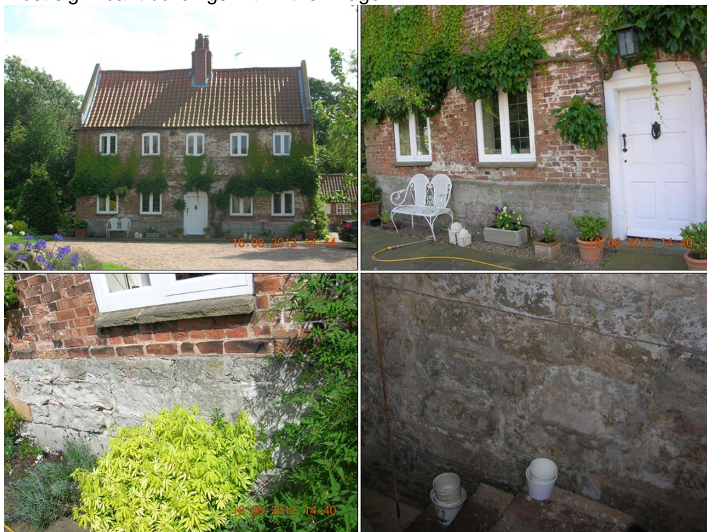
Figure 3.8: Views of Skerry Sandstone foundations at The Manor, including north elevation/frontage (top), east elevation (bottom left) and cellar (bottom right).
