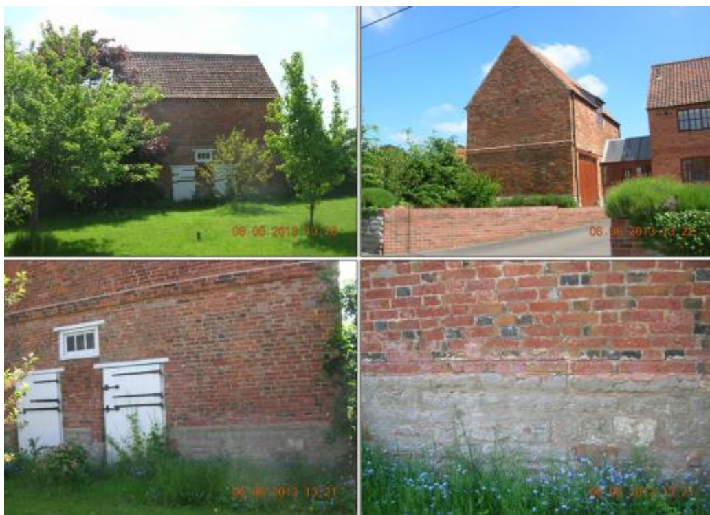
Figure 3.34: Former dovecote to Woodward Farm, showing earlier Skerry plinth (bottom), surviving timber joinery (left) and recent alterations as part of conversion to living accommodation and garage (top right).
