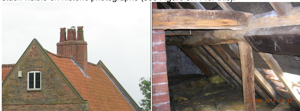
Figure 3.10: Steep roof pitch, central cross-plan chimney stack, raised and coped gables and internal roof timbers, all evidence of the 17 th century phase.
