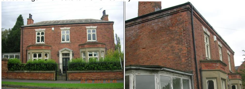
Figure 3.49: Views of Holly House, with join clearly visible on west elevation (right).
