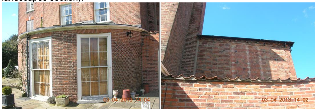
Figure 3.22: Early-19 th century bow (left) and first floor addition with Dearne's bond brickwork.
