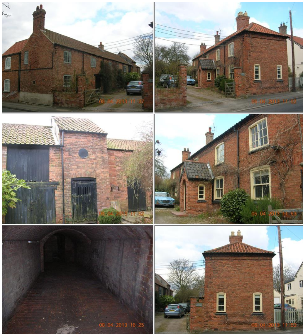
Figure 3.50: Views of The Old England (right) including the join in the brickwork clearly visible on the east elevation (bottom right); Views of the former brewery building adjacent to the house (left), including connecting tunnel between the two buildings (bottom left).
