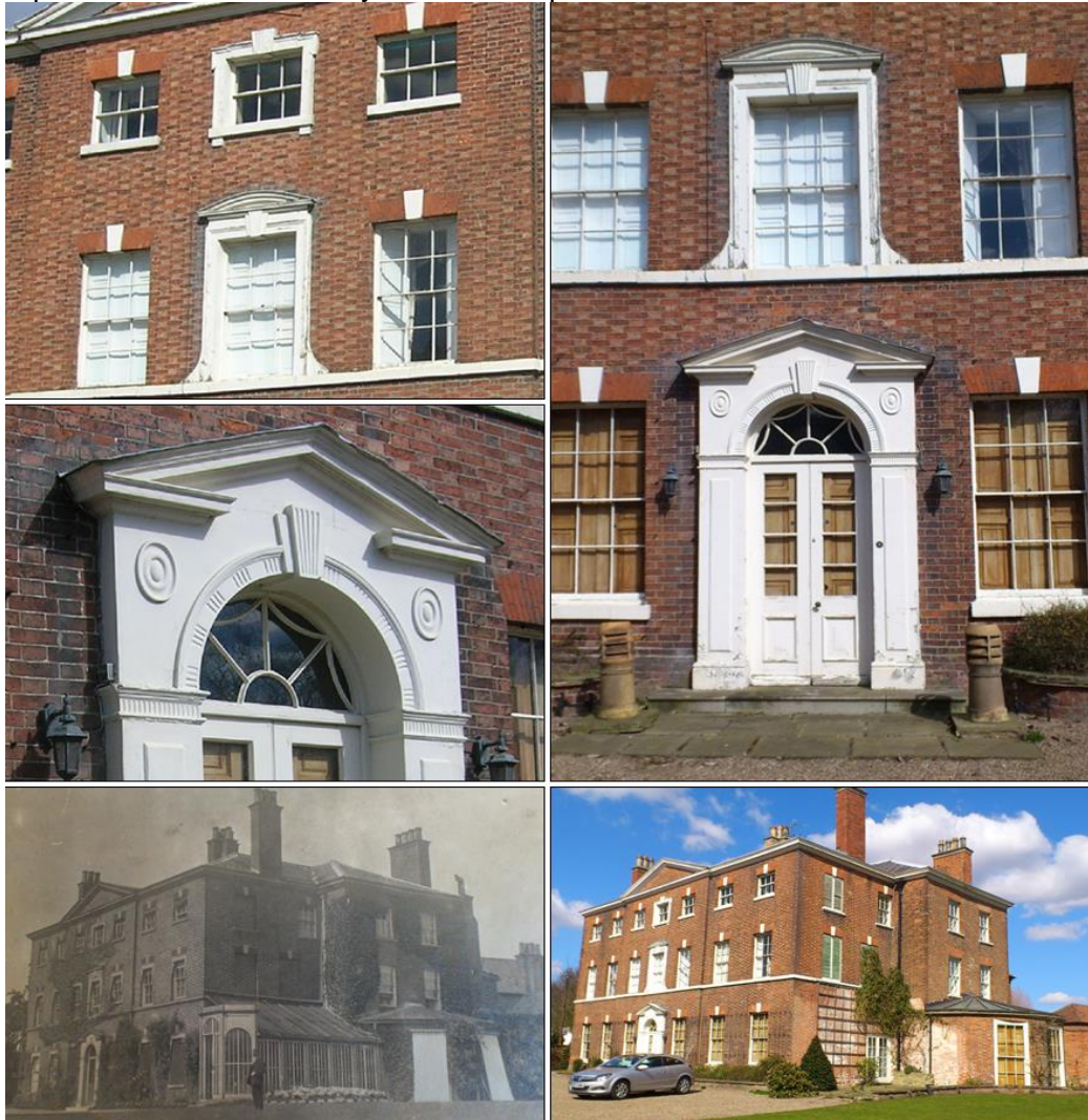
Figure 3.20: Main c1777 façade of East Markham House, including decorative doorway with paterae, pediment and traceried fanlight (centre left), first floor window (top right), second floor window (top left) and comparative views from c1909 (bottom left) and present day (bottom right). Image source: East Markham Hall owners, accessed 2013.
