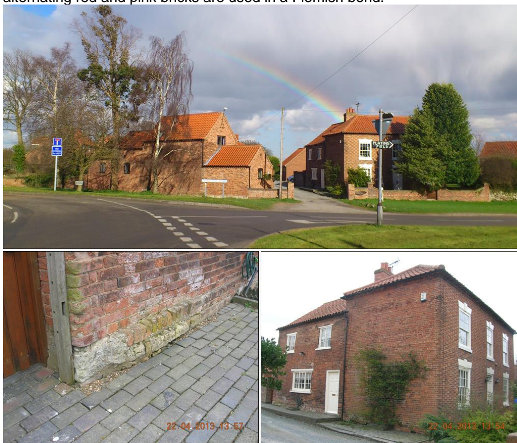
Figure 3.29: Pond Farm (top), with earlier Skerry Sandstone foundations (bottom left) and distinction between 18 th and 19 th century portions (bottom right).
