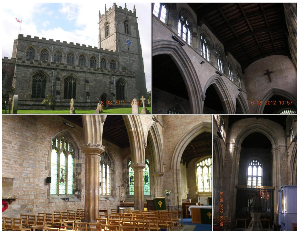
Figure 3.5: Views of church, showing north face of nave (top left), internal side of nave clerestory window openings (top right), octagonal columns within the nave (bottom left) and high arch through to the western tower (bottom right).
