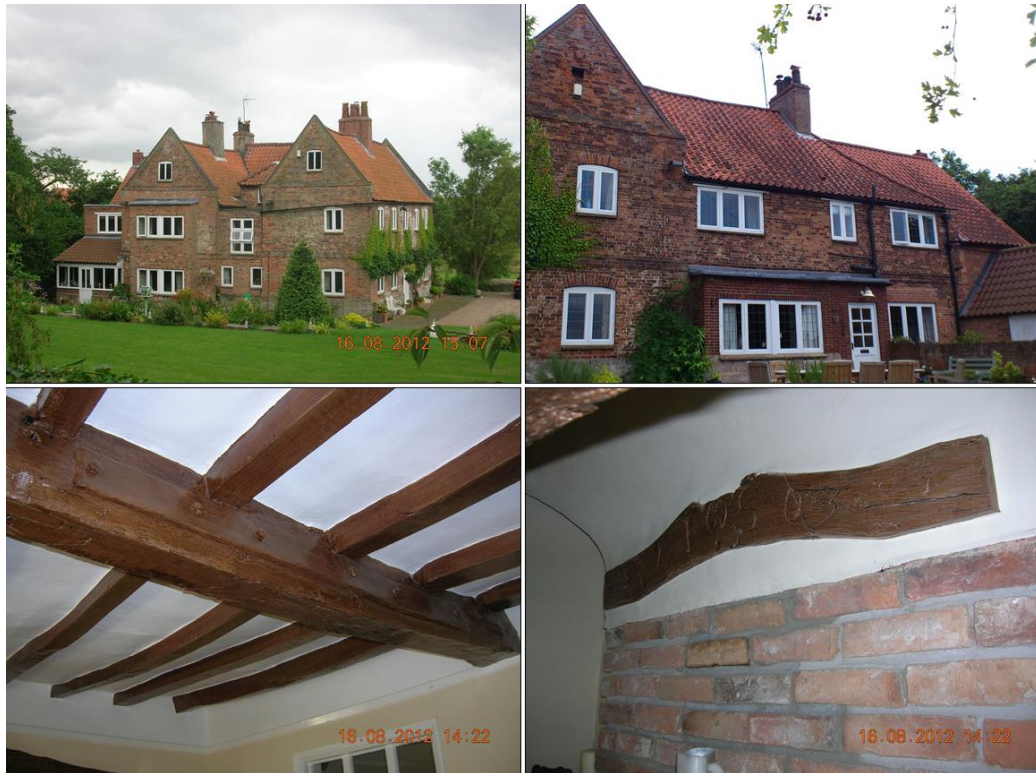
Figure 3.9: Evidence of 17 th century plan form and construction, including external views of 2 ½ storey elements from north east (top left) and north west (top right), with internal 17 th century timber beams supporting first floor (bottom left); timber beam with “1703” inscription on ground floor (bottom right).
