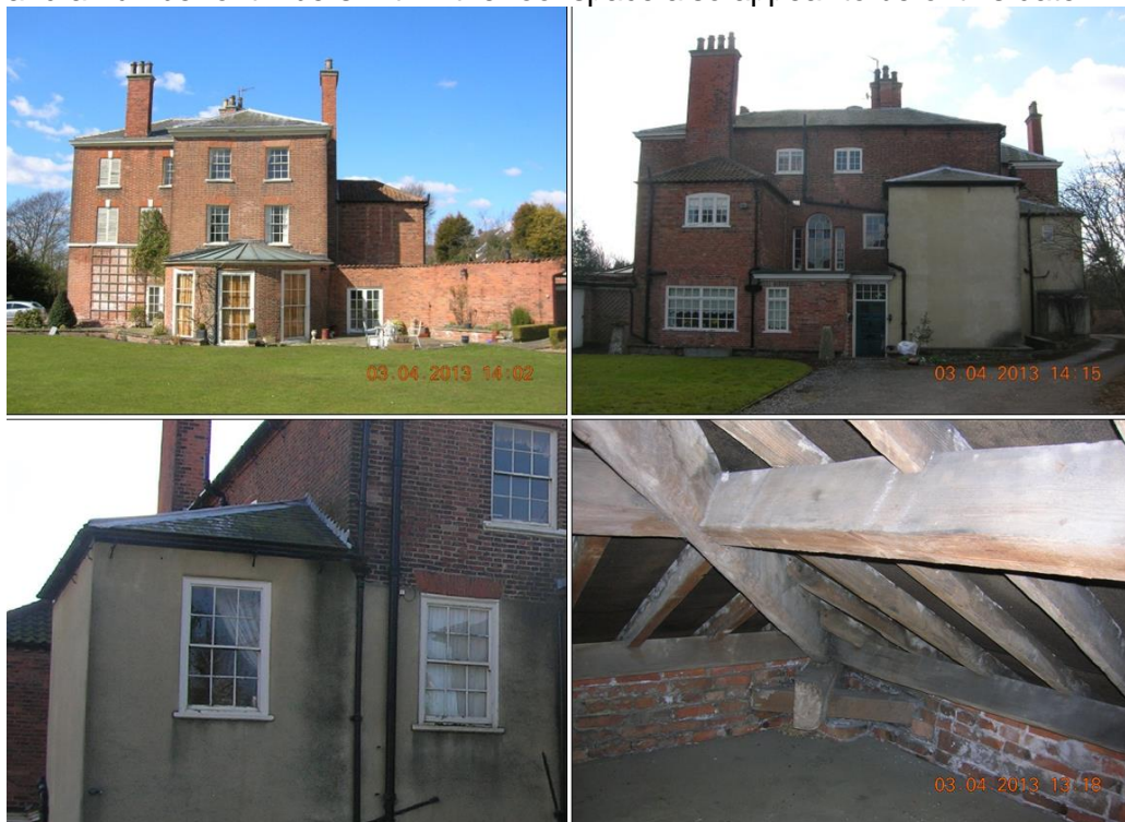
Figure 3.18: Early-18 th century features at East Markham Hall including the quadripartite chimney stack (top), the flush-fitting sash on the north west side (bottom left) and the dragon beams in the roof space (bottom right).
