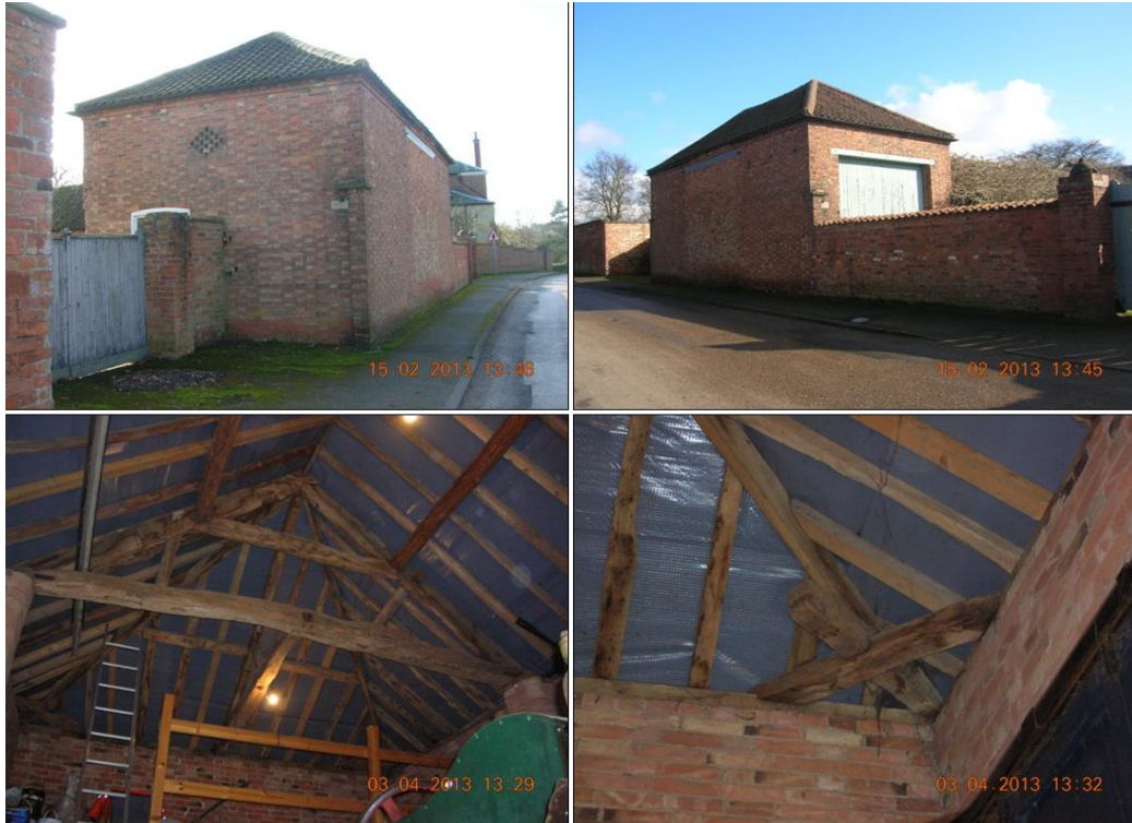
Figure 3.23: Late-18 th /early-19 th century barn with 17 th century timber roof structure. The distinctive dragon beams (bottom right) exist in each of the four corners.
