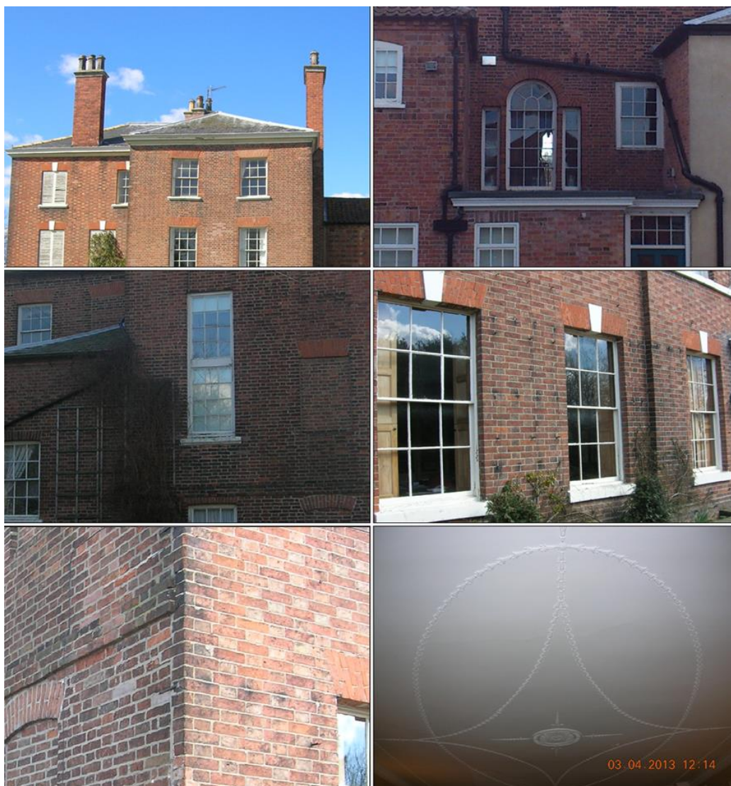
Figure 3.21: Other significant features from the c1777 phase, including the tall chimney stacks (top left), Palladian window (top right), remodelled window heads (centre left), deeply-recessed sashes (centre right), the join between the c1701 building and the c1777 façade (bottom left) and decorative internal plasterwork (bottom right). The centre left image also shows an early-18 th century brick arch, which uses rectangular bricks and thicker mortar joints at the top.
