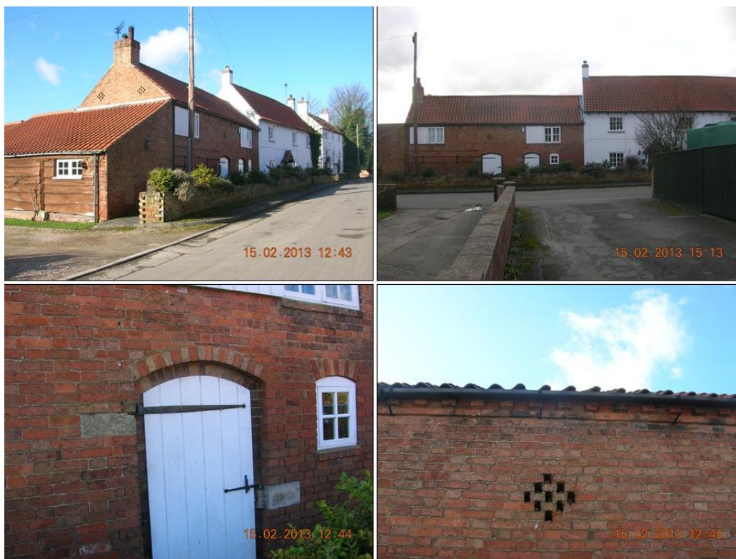
Figure 3.42: Views of 19 th century stable building at Whitehouse Farm, including alternating brick arch (bottom left) and diamond ventilator (bottom right).
