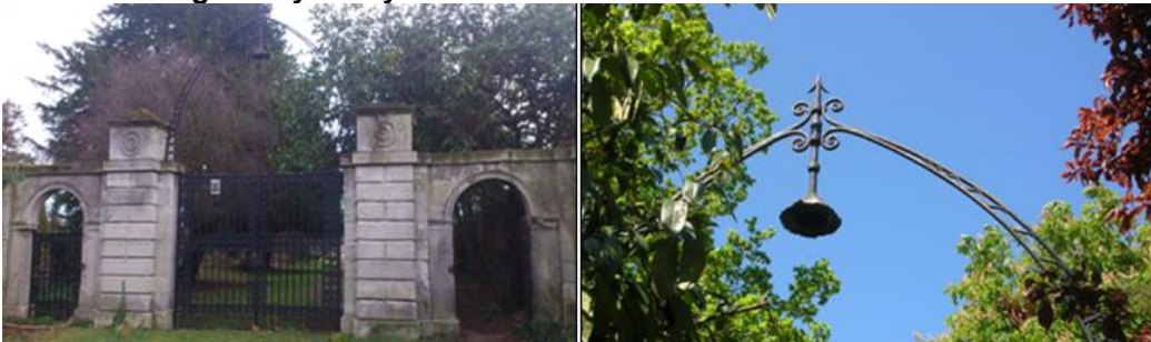
Figure 4.2: Stone has deteriorated, particularly around the metal mounting joints. The light is also missing and the iron fitting is damaged.
