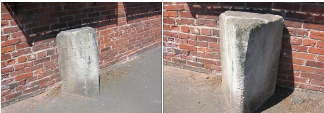
Figure 4.3: Stonework has deteriorated considerably; much of the inscription is no longer legible.
