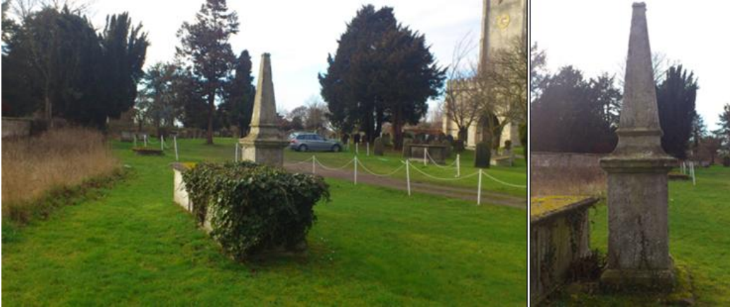
Figure 4.1: Top of monument is damaged, stonework has deteriorated, much of the inscription is no longer legible. Adjacent associated tomb is also in considerable disrepair, with cracks, vegetation growth and erosion of stonework.
