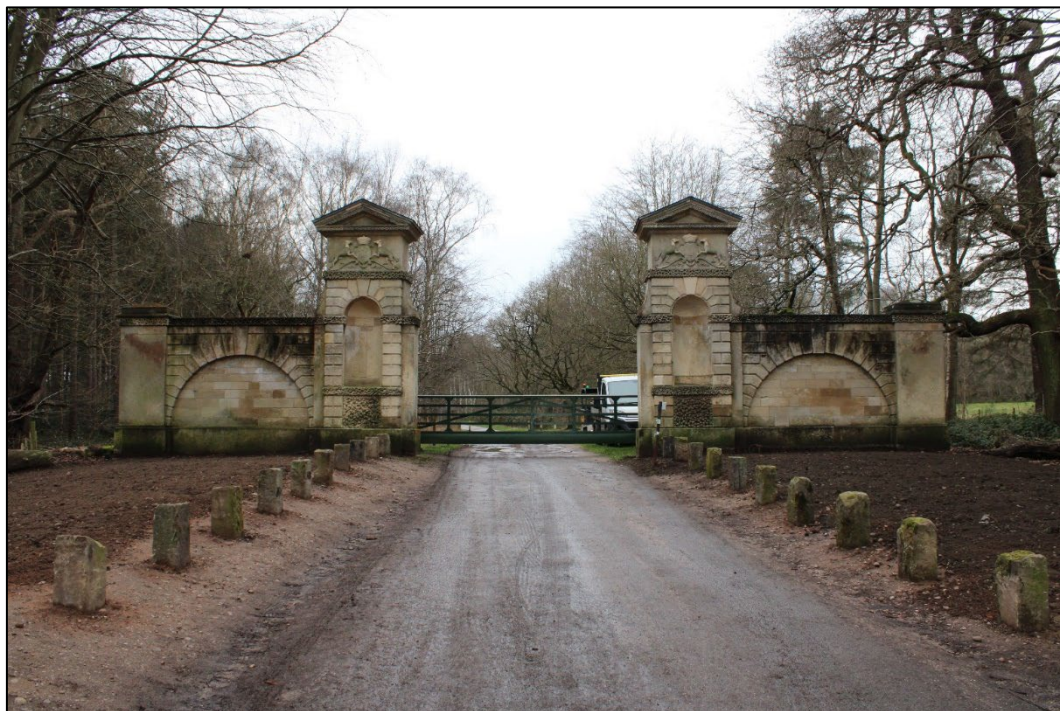
Plate 5: Grade II* Listed Drayton Gate (NHLE: 1045058)
