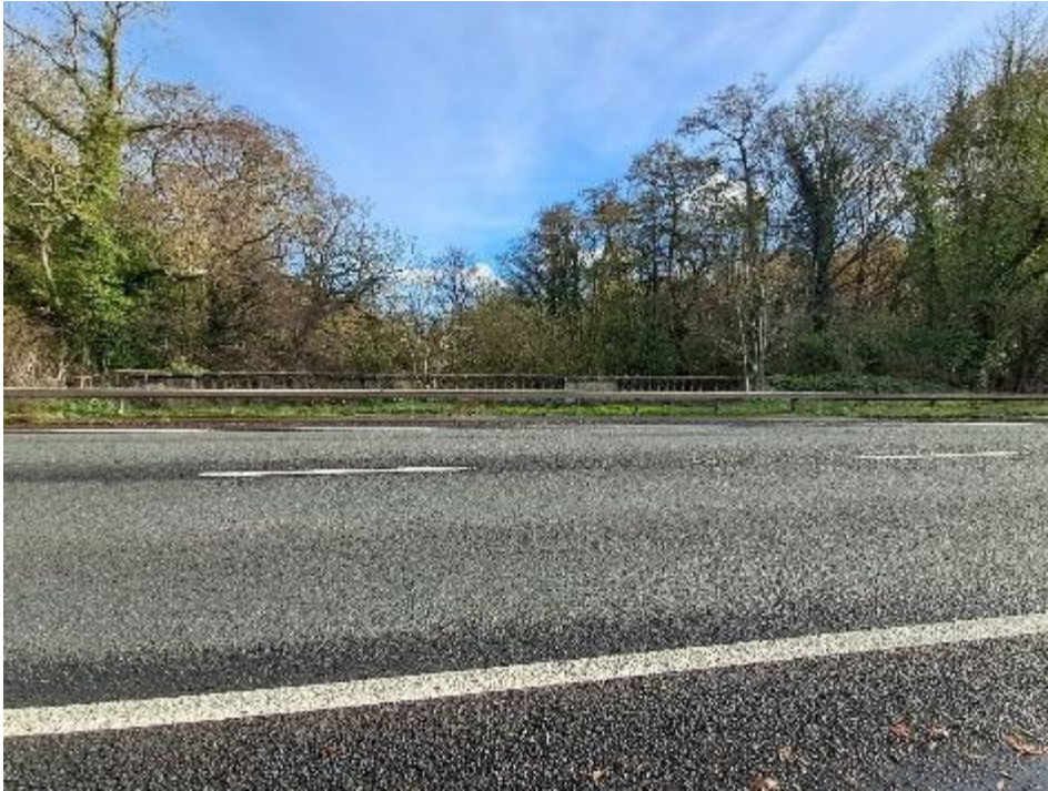
Plate 19: West Bridge looking to east
